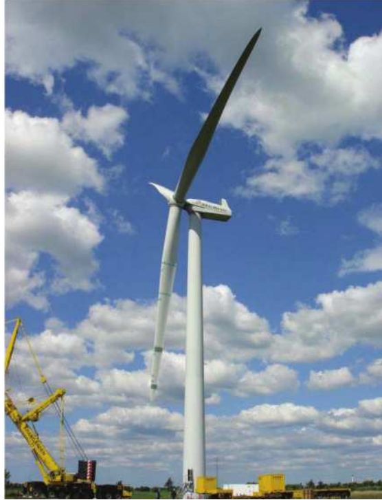
Fig. 1 The NM80 wind turbine in Tjæreborg
