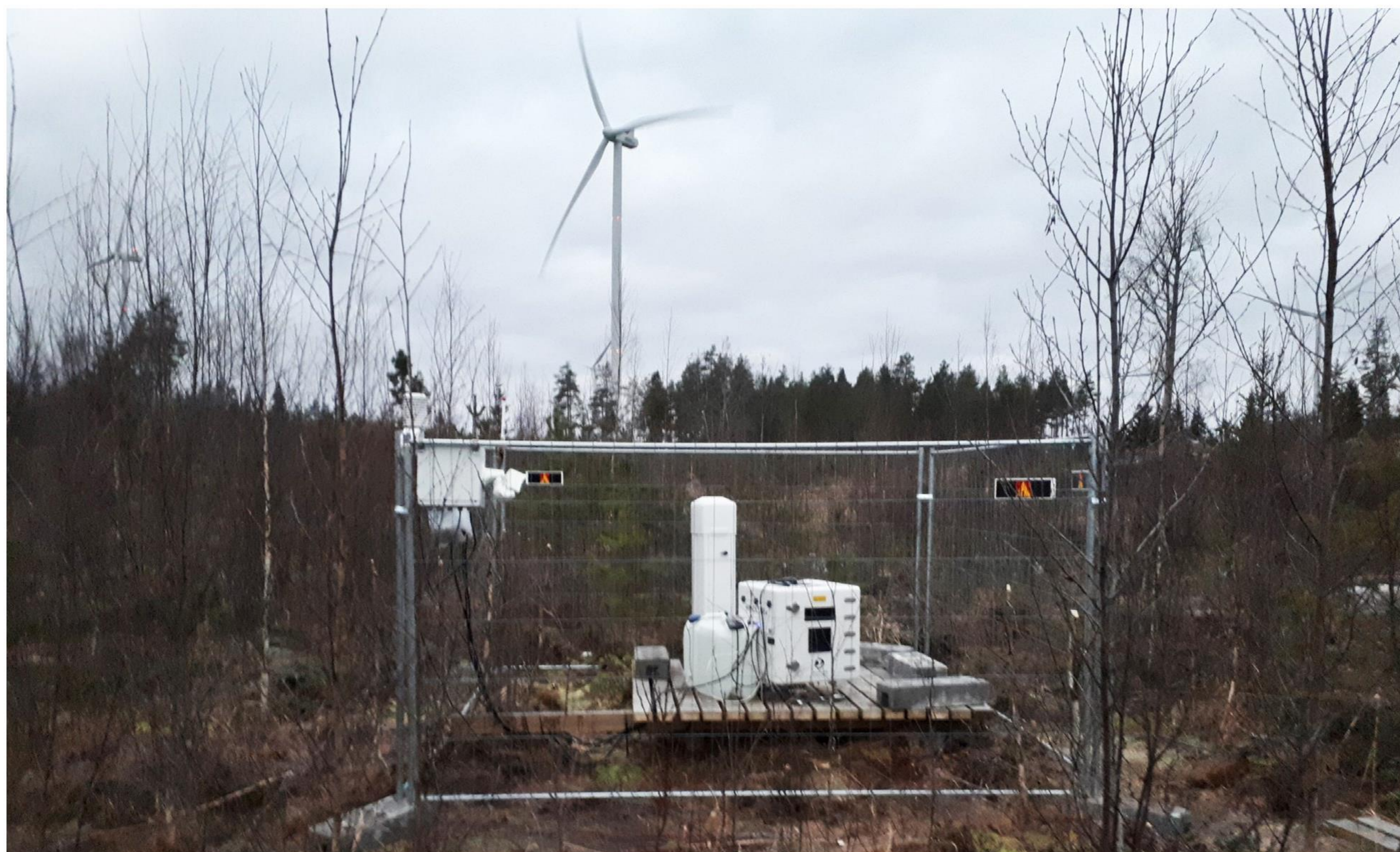
FIGURE 4 COMBINED MEASUREMENTS OF WIND, ATMOSPHERIC DATA, AND BLADE LOADS ARE KEY TO BETTER MODELLING OF INFLOW AND WAKES, AND ONE OF THE KEY OUTCOMES OF ONGOING TUTTE PROJECT (2020-2022). THE PICTURE SHOWS ONE OF THE MEASUREMENT STATIONS IN TUTTE INSTALLED IN A FINNISH WIND FARM (SOURCE VTT).
