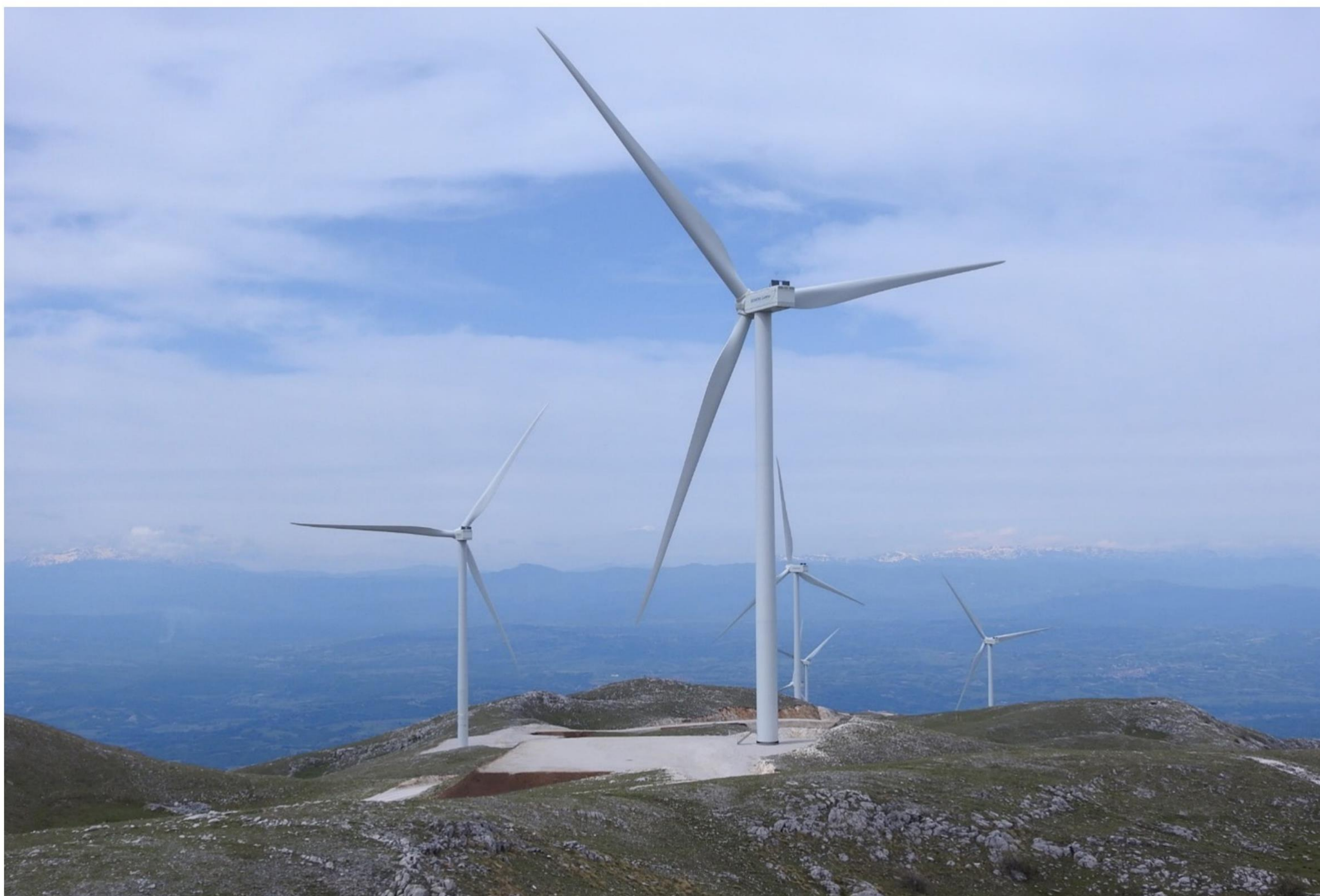
WIND FARM IN WEST MACEDONIA, GREECE (SOURCE: CRES)
