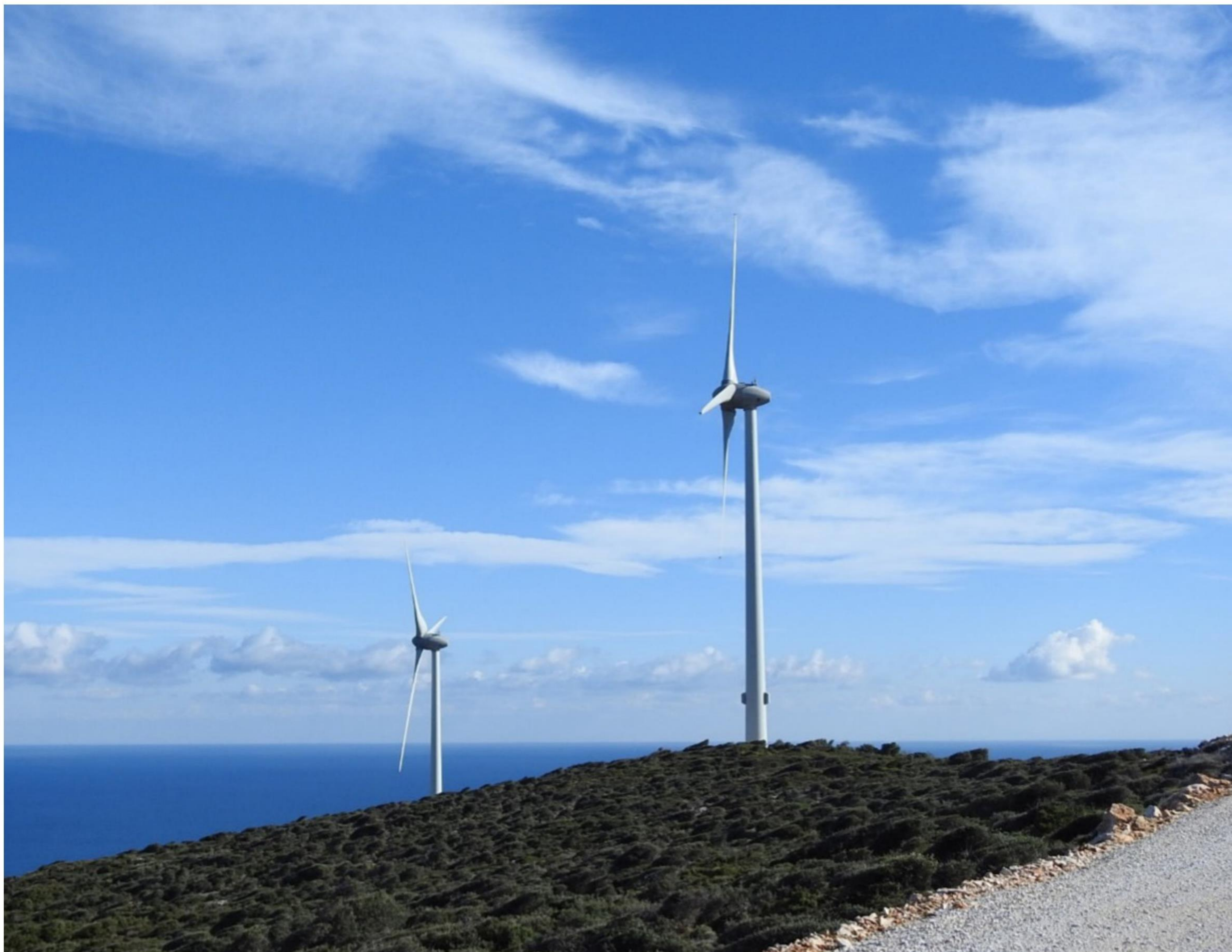
WIND FARM IN EVIA, CENTRAL GREECE (SOURCE: CRES)
