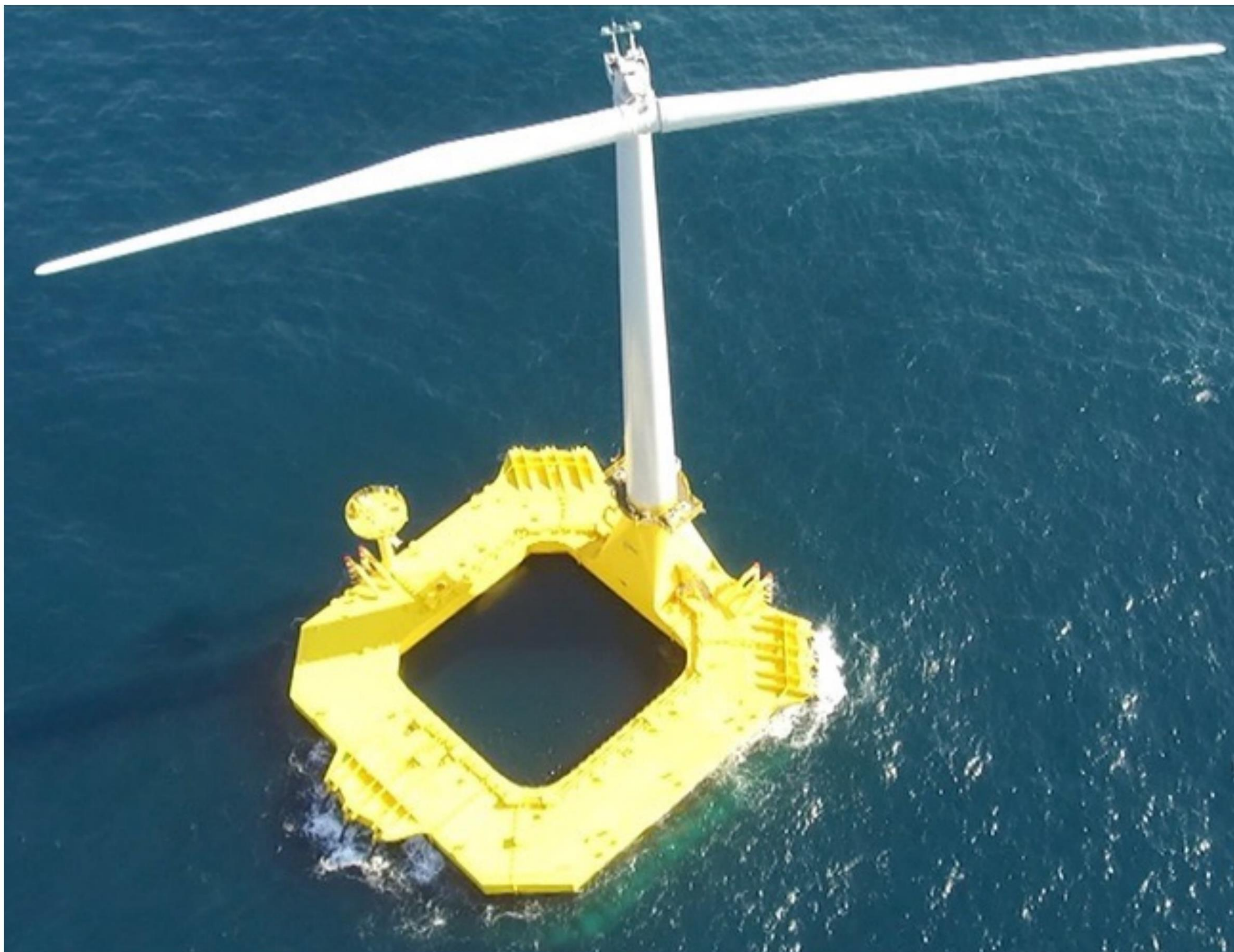
FLOATING FORM WIND TURBINE HIBIKI MANUFACTURED BY HITACHI ZOSEN CO., LTD., INSTALLED 15 KILOMETERS OFFSHORE OF KITAKYUSHU CITY.
