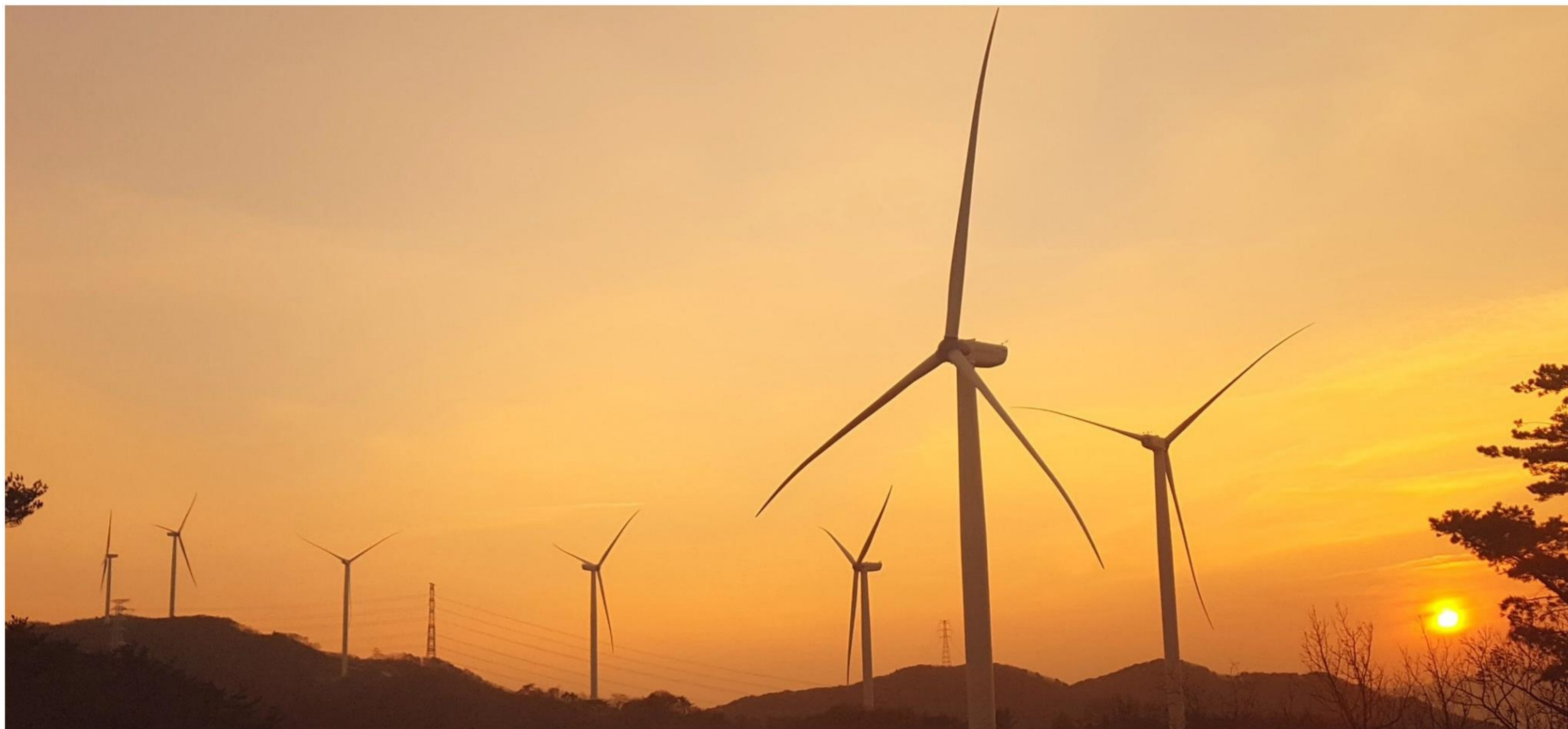
[PHOTO 2] GYEONG-JU WIND FARM, GYEONGSANGNAM-DO, KOREA, UNISON 2.3MW WTG, SOURCE: UNISON CO., LTD.
