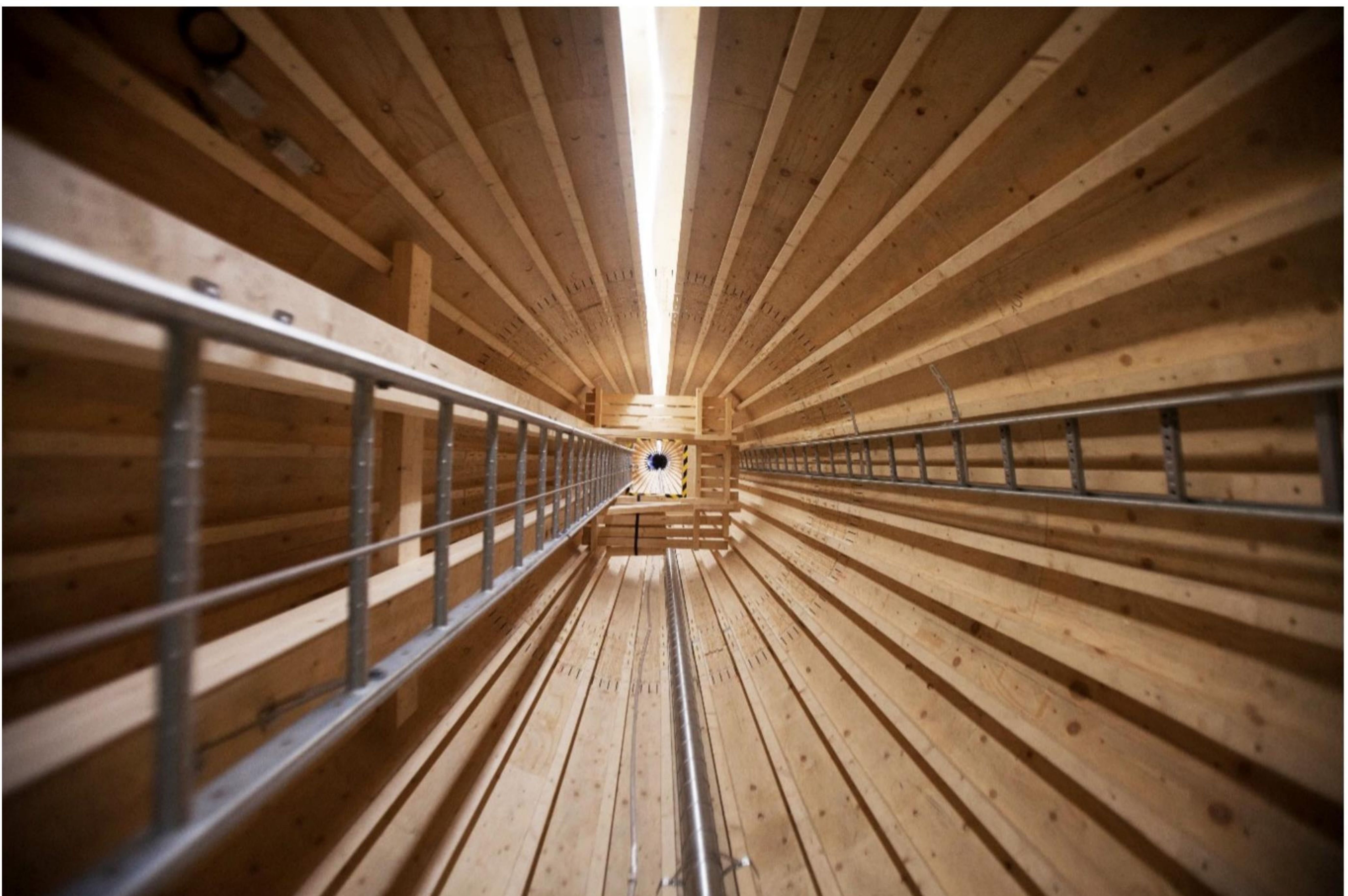
INSIDE VIEW OF THE 30 M WOODEN TURBINE TOWER FROM MODVION ON BJÖRKÖ (GOTHENBURG) (SOURCE: MODVION).
