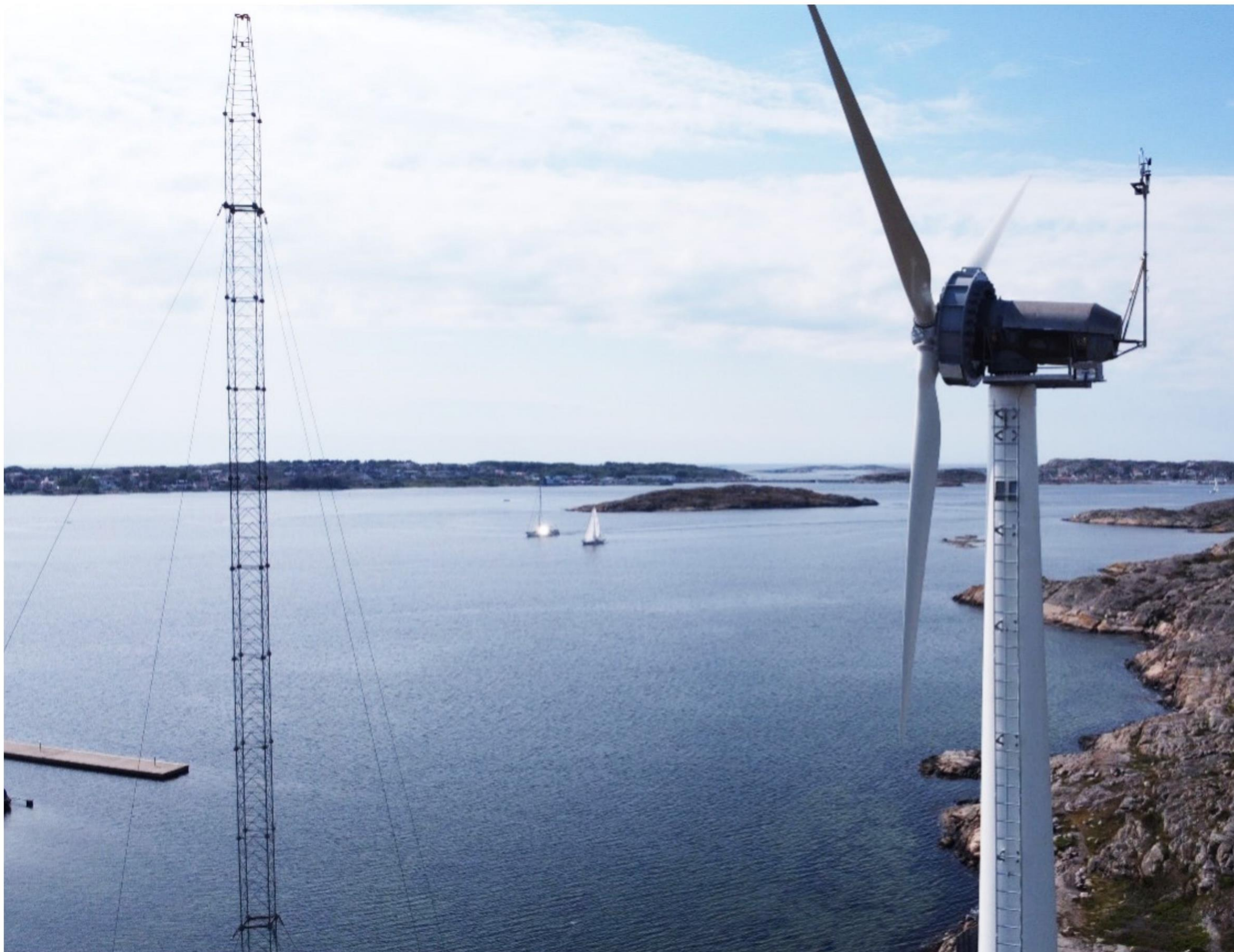
PROTOTYPE TURBINE AT SWPTC WITH WOODEN TOWER FROM MODVION ON BJÖRKÖ (GOTHENBURG), NACELLE HEIGHT 30 M, ROTOR DIAMETER 16 M. (SOURCE: MODVION).
