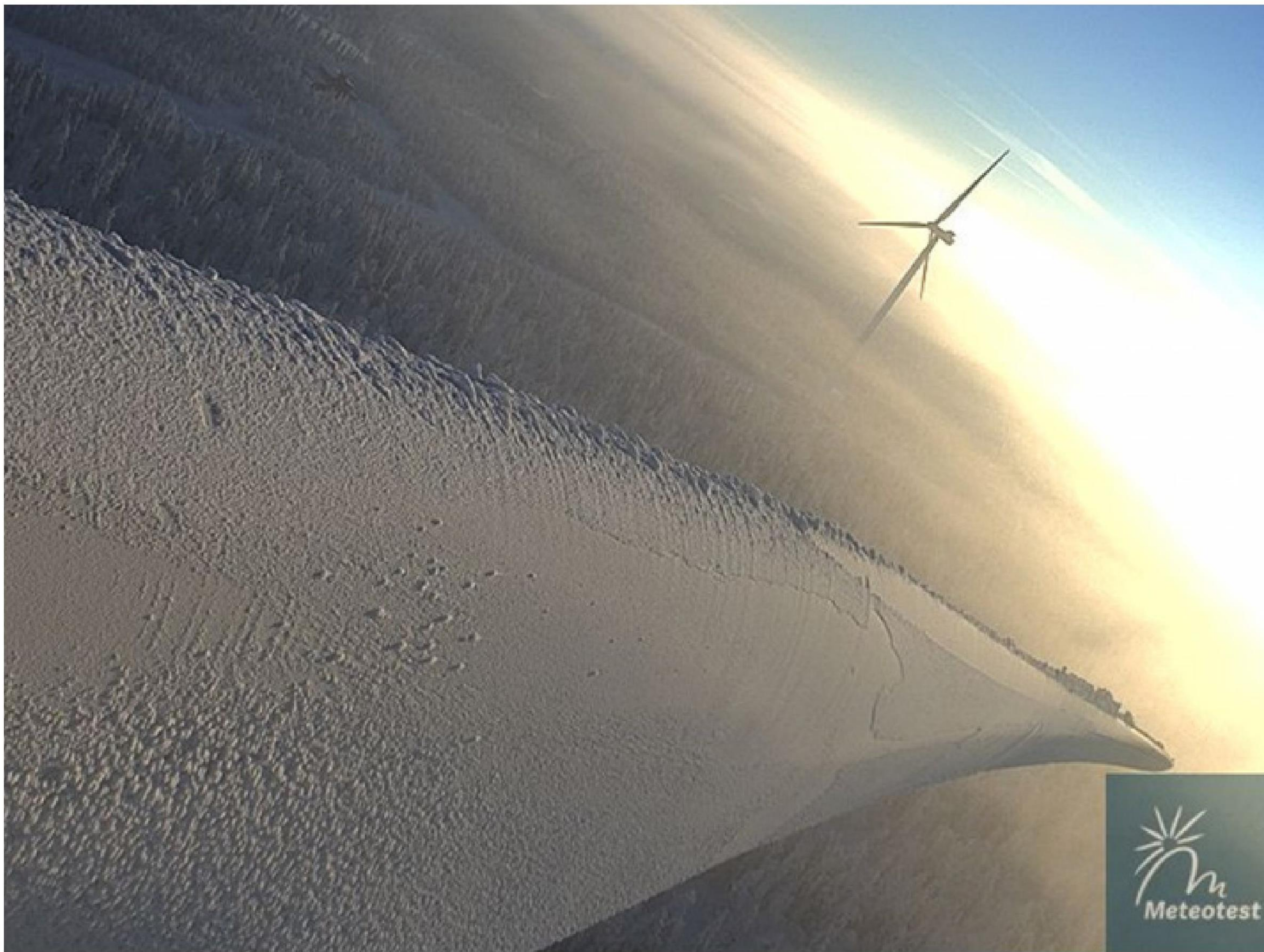
RIME ICE ON A WIND TURBINE BLADE. PICTURE COURTESY OF METEOTEST
