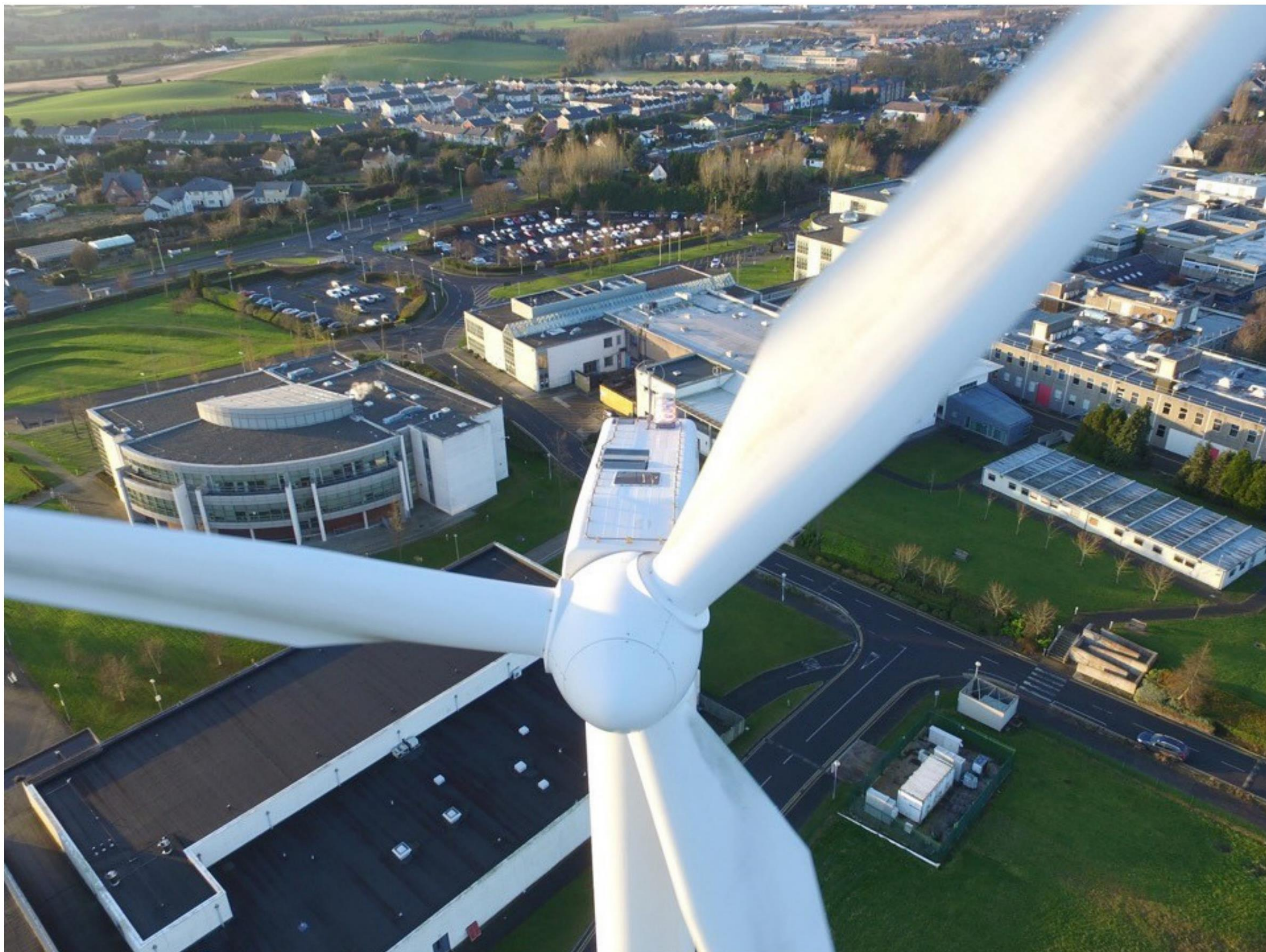
CAPTION: THIS 850-KW VESTAS V52 IS ON THE CAMPUS OF THE DUNDALK INSTITUTE OF TECHNOLOGY. TASK 41 RESEARCHERS HAVE USED ITS OPERATIONAL DATA FOR COLLABORATIVE RESEARCH AND PUBLICATIONS. PHOTO CREDIT: RAYMOND BYRNE, DUNDALK INSTITUTE OF TECHNOLOGY
