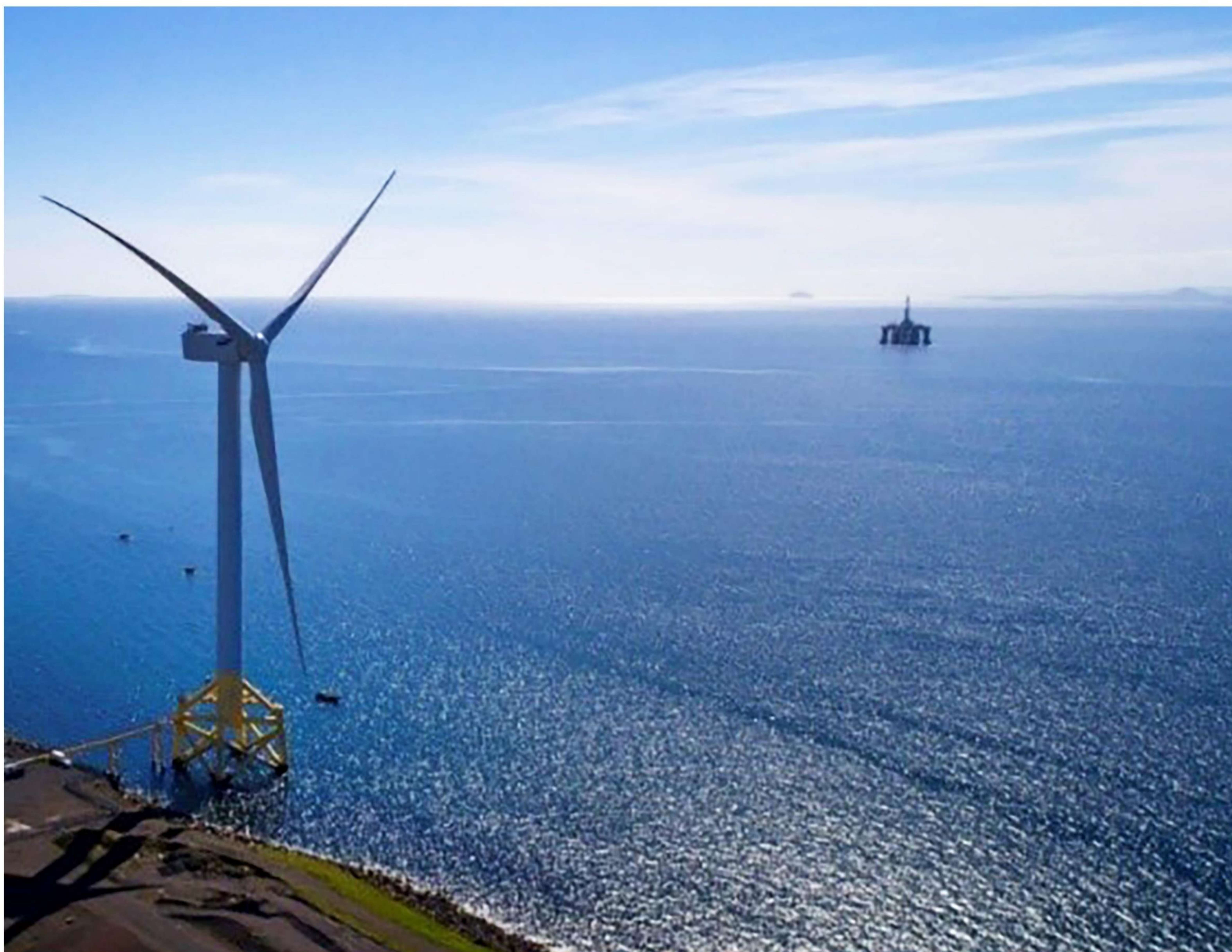
7 MW LEVENMOUTH DEMONSTRATION TURBINE (SOURCE: ORE CATAPULT)
