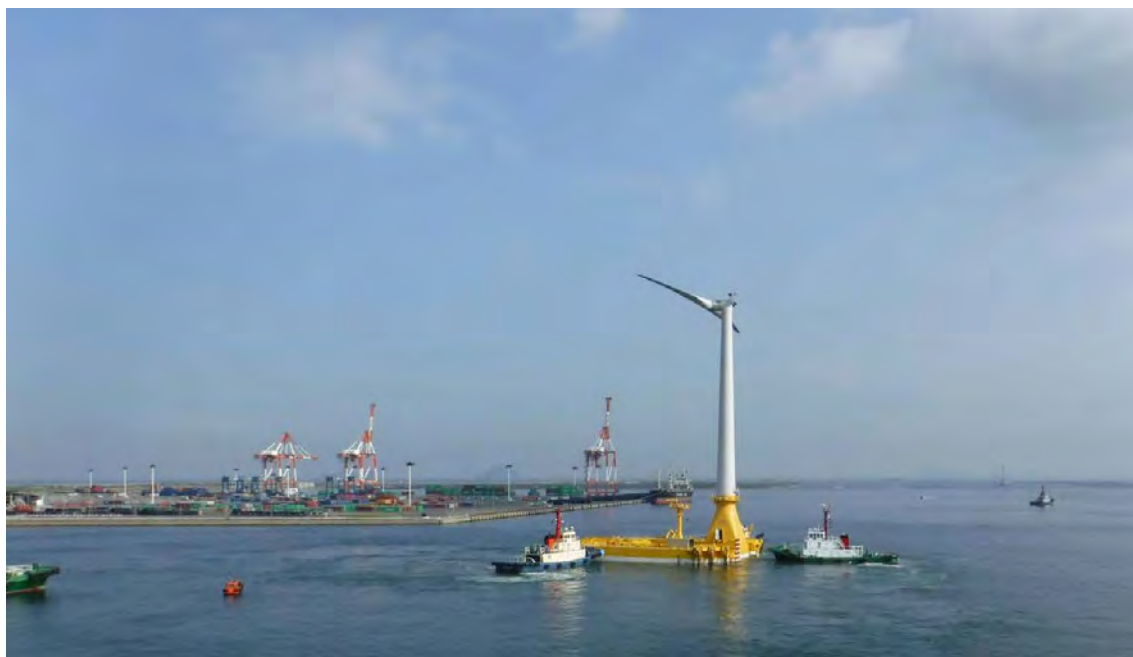
Figure 3. Offshore floater and turbine system being towed by tugboats
