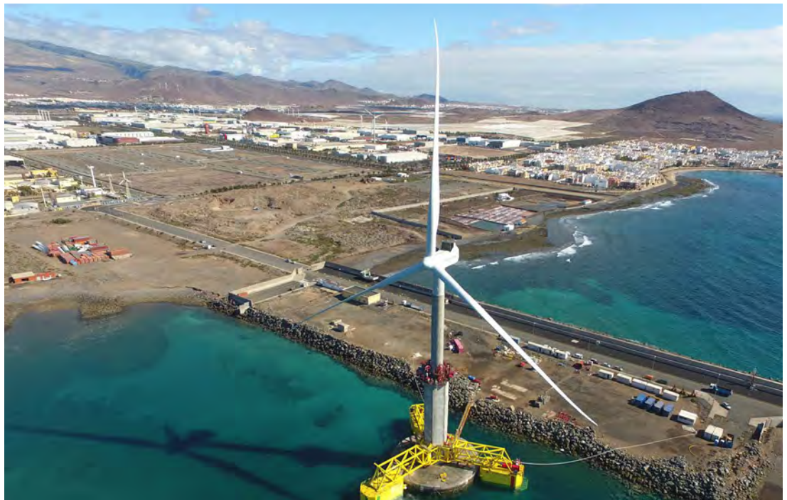
Figure 11. The ELISA-ELICAN Project, a 5-MW offshore wind turbine installed in Gran Canaria Island (Spain). The project features a self-installing precast concrete telescopic tower and foundation. This was the first bottom offshore wind turbine installed without using a heavy-lift vessel. (Photo credit: ESTEYCO)
