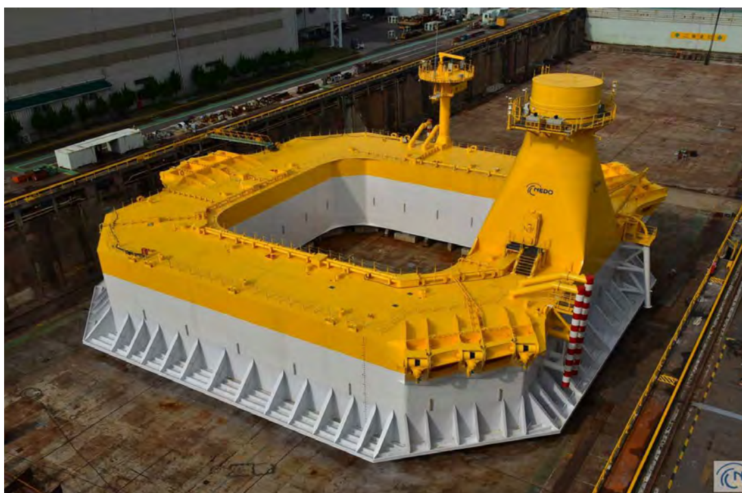
Figure 2. Offshore floater under construction at Hitachi Zosen (barge type)
