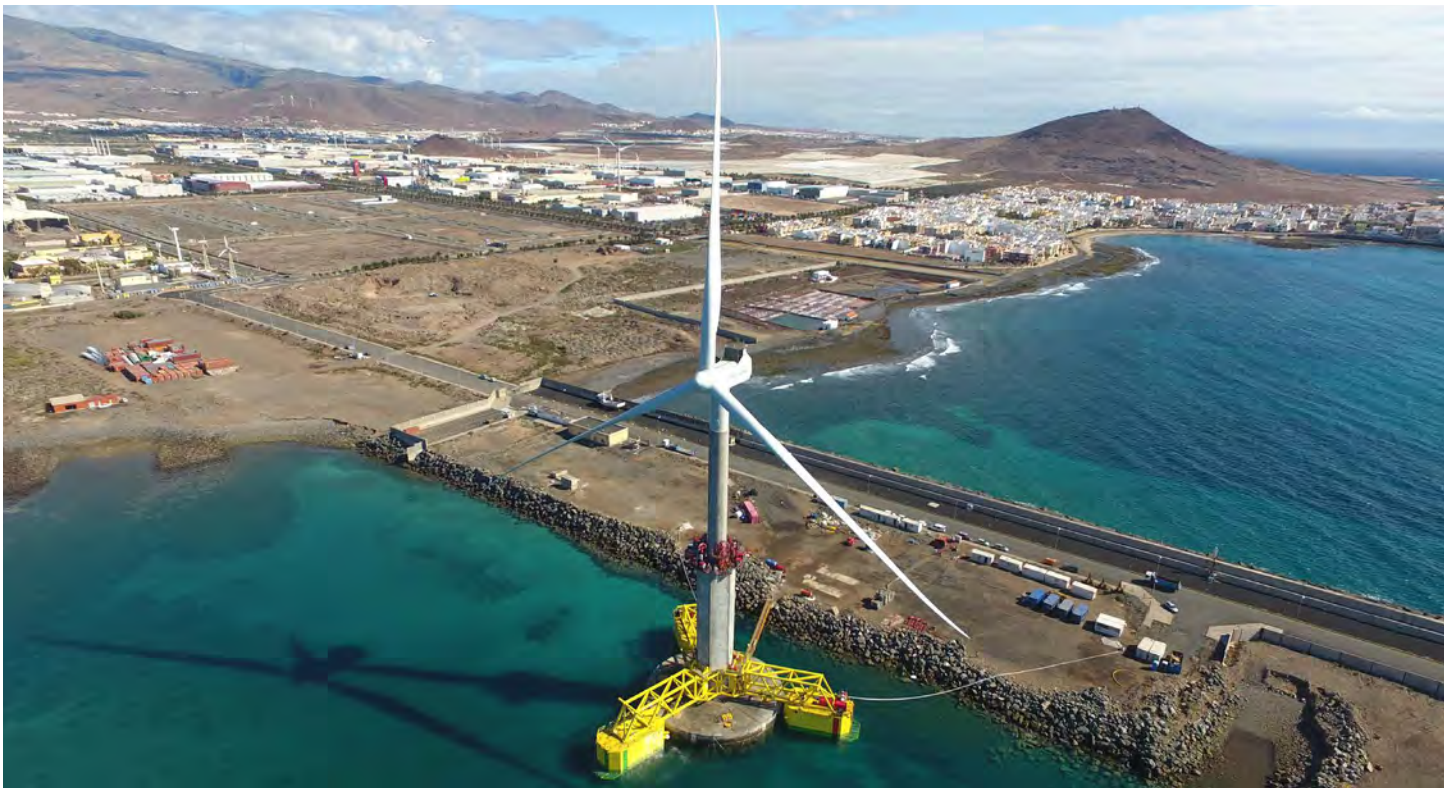
Figure 3. ELISA-ELICAN Project: A 5-MW offshore wind turbine installed in Gran Canaria Island, Spain. Self-installing precast concrete telescopic tower and foundation; the first bottom offshore wind turbine ever installed with no need for heavy-lift vessels. (Photo credit: ESTEYCO)
