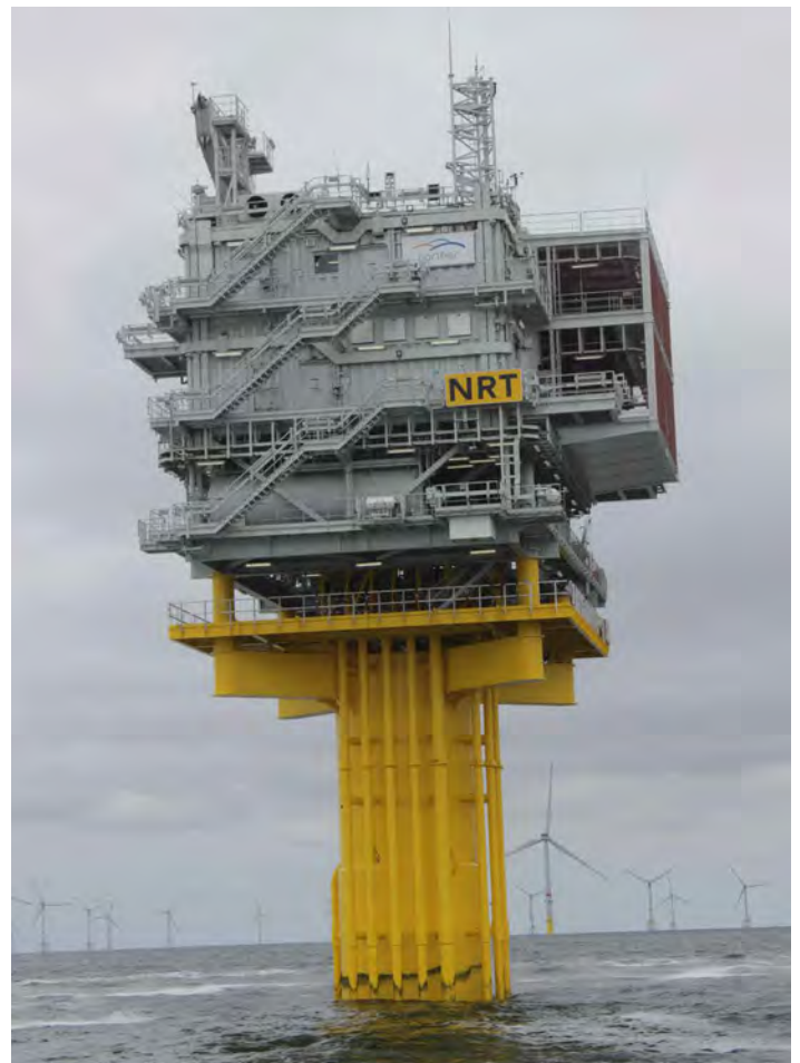
Figure 2. Belgian offshore wind farm in the North Sea
