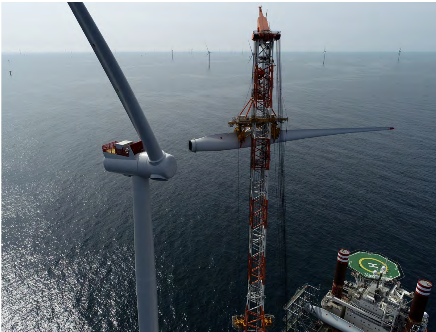
INSTALLATION OF SIEMENS GAMESA 7MW TURBINE AT HORNSEA ONE (PHOTO: ØRSTED)
