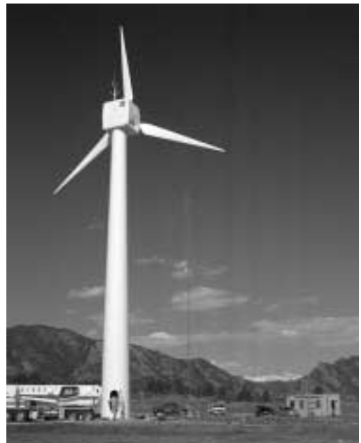
Figure 21.6 Northern Power Systems' 100-kW cold weather turbine undergoing field tests at the National Wind Technology Center in Colorado and operational tests in Kotzebue, Alaska
