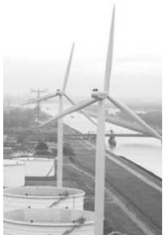
Figure 14.3 2.5-MW wind turbines at Nerefco refinery
