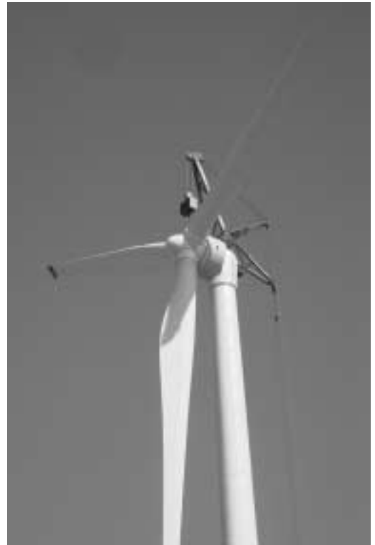
Figure 14.4 Erection of Lagerwey 1.5 to 2 MW prototype
