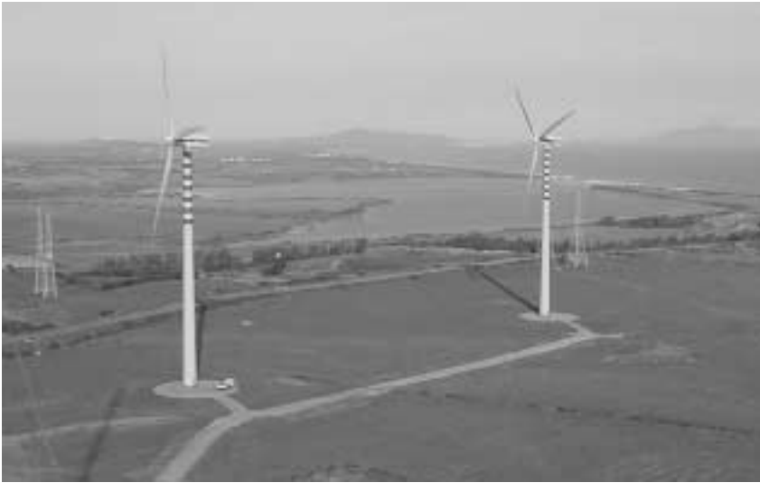
Figure 11.6 Enel GreenPower's 12.25-MW wind farm, with seven Vestas V-66 units of 1,750 kW, at Alta Nurra site, in Sardinia
