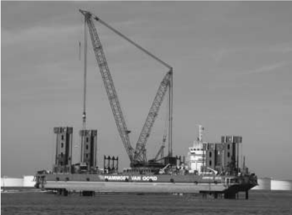
Figure 14.5 Jumping Jack offshore installation barge
