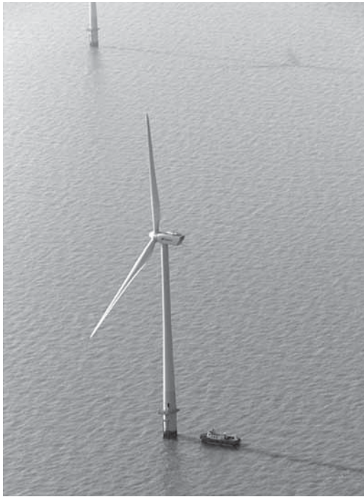
Figure 1 One of the thirty 3-MW turbines at Kentish Flats Offshore Wind Farm (Photo courtesy of Elsam A/S).
