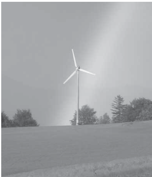
Figure 5 Aventa AV 7: Swiss-made wind turbine for low wind speeds.
