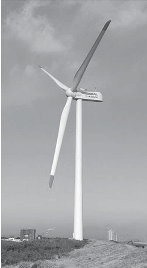
Figure 5 FHI's new 2-MW, down-wind type wind turbine, the SUBARU 80/2.0, installed at Hazaki.
