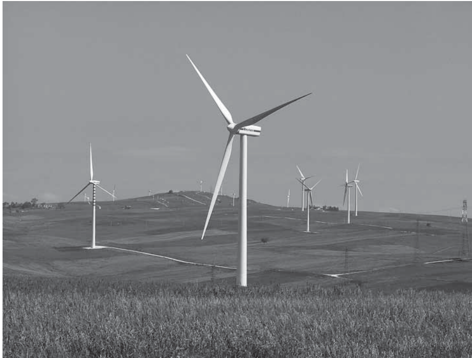
Figure 5 At the end of 2005, Italy enjoyed more than 1.7 GW of total installed wind capacity including these 2-MW Vestas V80 turbines of FRI-EL in the Campania region.
