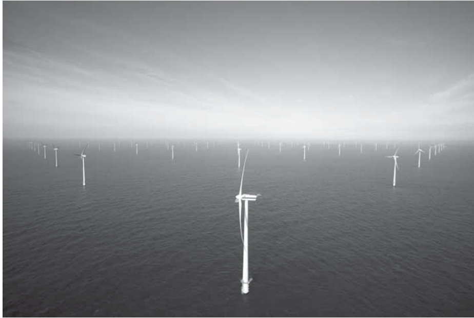
Figure 6 Offshore wind farm at Horns Rev, 160 MW. Published with the permission of ELSAM.
