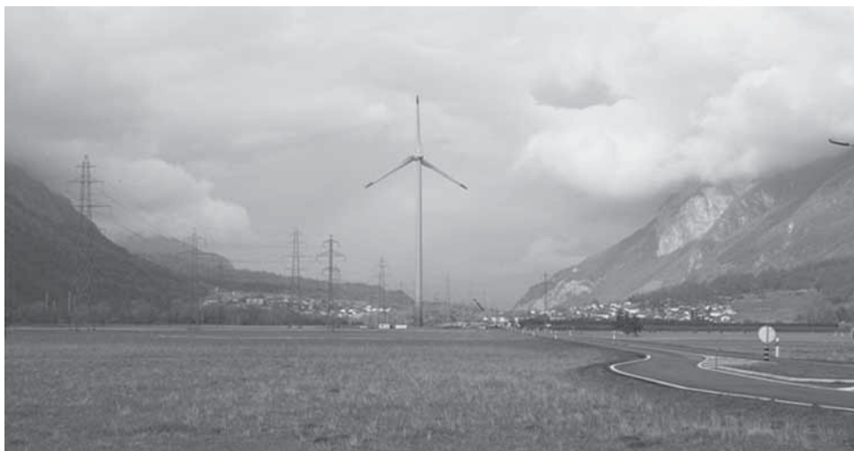
Figure 7 The 2-MW wind power plant in Collonges, canton Valais.
