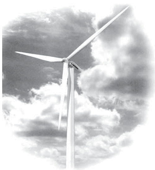
Figure 4 MHI's new 2.4-MW wind turbine, the MWT92, installed in Yokohama.
