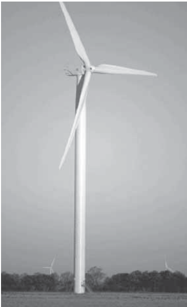
Figure 4 GE Energy's 2.5xl wind turbine has a 100-meter rotor and operates at sites with average wind speeds of up to 8.5 mps.
