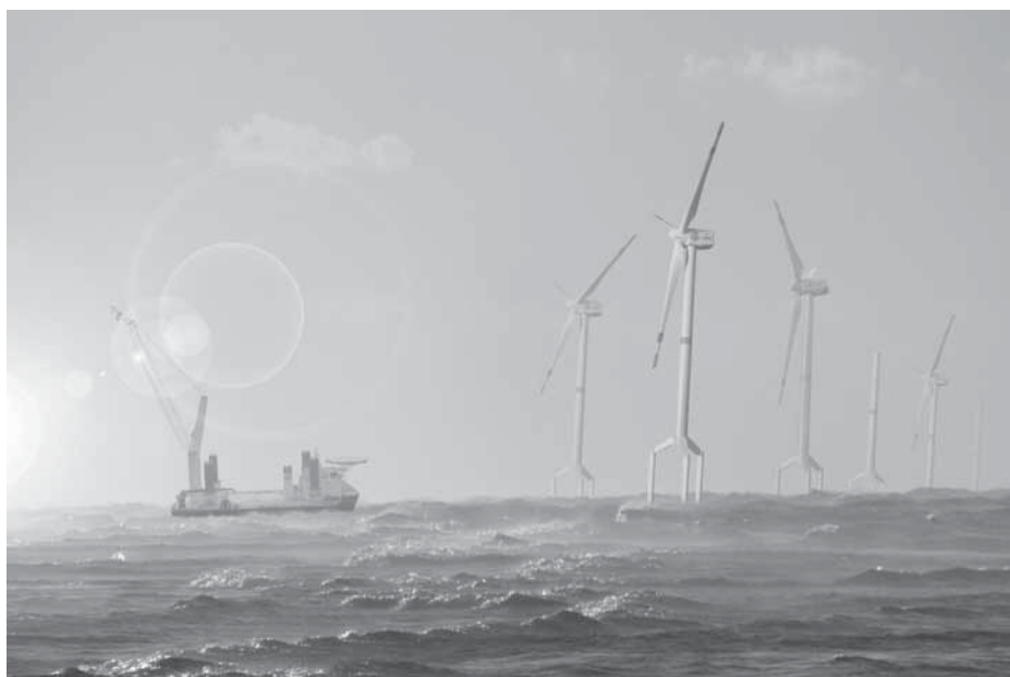
Figure 8 Animation of BARD's construction of an offshore wind farm with VM, "Wind Lift I" and tri-pile foundations, BARD Engineering GmbH.
