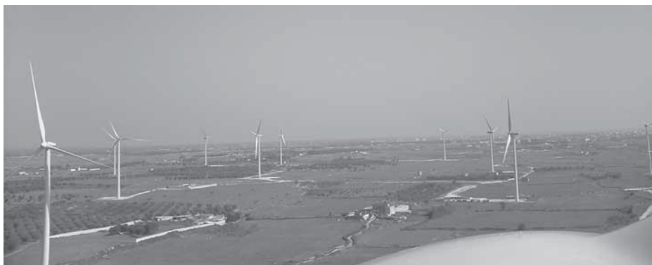
Figure 6 Vestas V90 turbines at the 36-MW Surbo wind farm developed by Inergia in Apulia (courtesy of Vestas).
