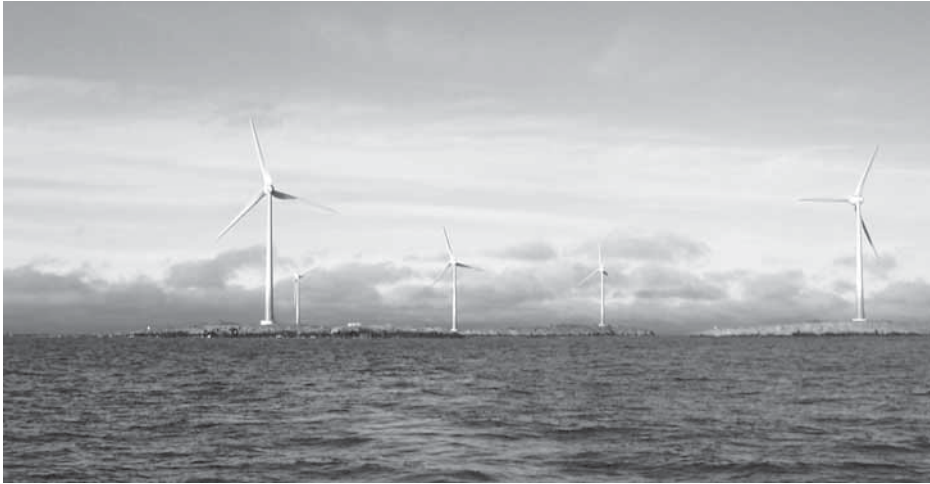
Figure 3 New semi-offshore wind farm (6 x 2.3 MW) installed on the cliffs and small islands in Åland archipelago, Båtskäär (Photo: Henrik Lindqvist).
