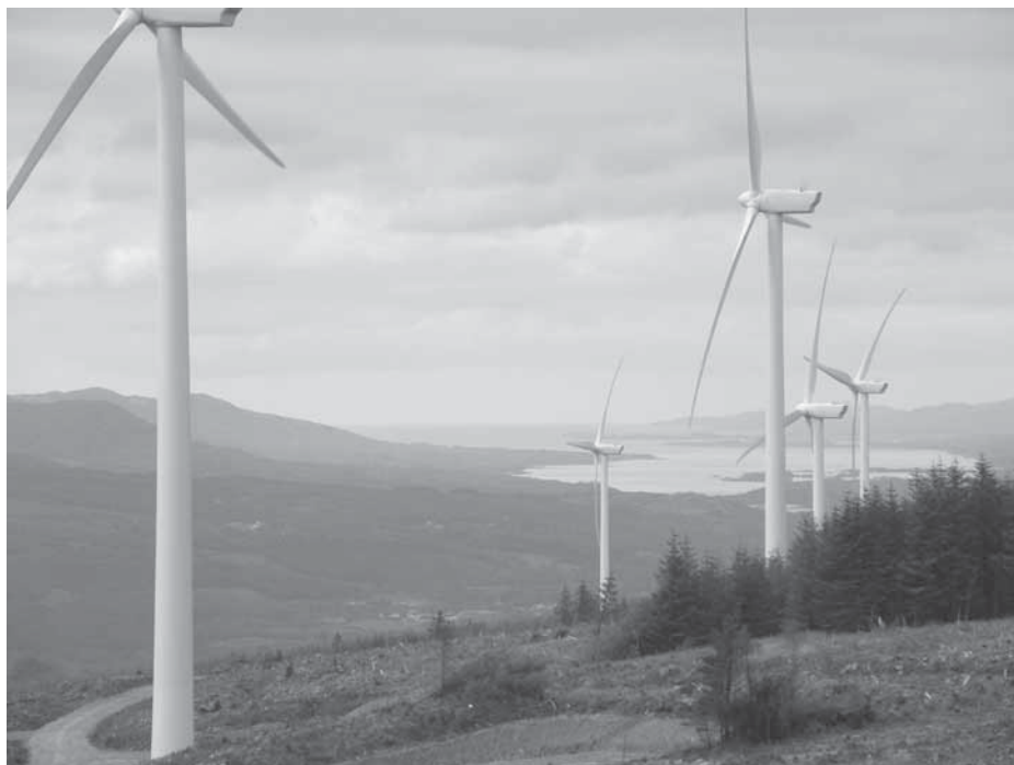
Figure 2 Kilgarvan Wind Farm with 3-MW Vestas V90 turbines. Photo credit: TJ Hunter SWS Natural Resources.
