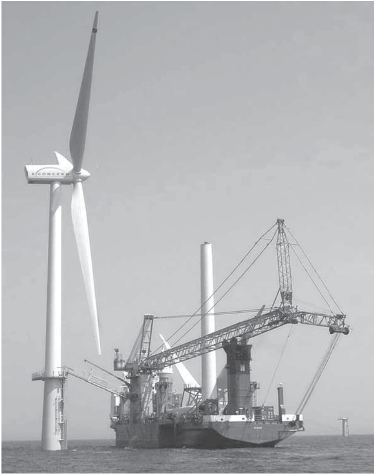
Figure 1 Q7 Offshore Wind farm installation of turbines. Photo Econcern
