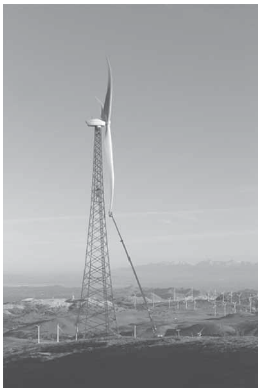
Figure 6 Knight and Carver's STAR blade installed on a Zond Z-48 wind turbine in Tehachapi, California for testing in 2008.
