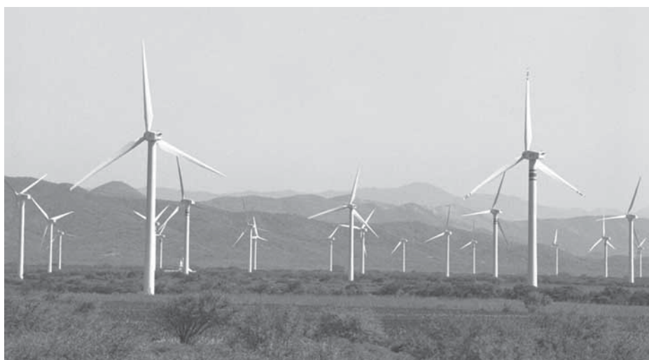
Figure 2 La Venta II 83.3-MW windfarm on the Isthmus of Tehuantepec, Mexico.
