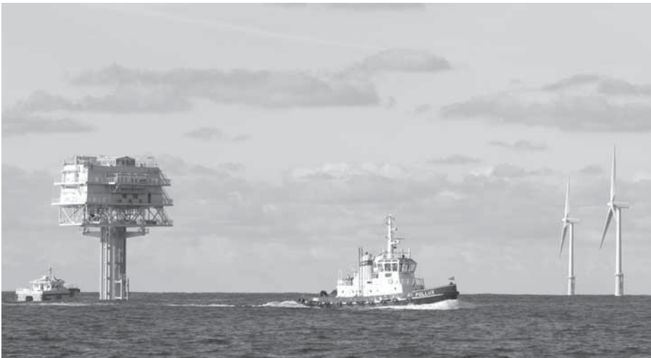
Figure 7 Q7 Wind Farm turbines and transformer station on monopile. Photo: Econcern.
