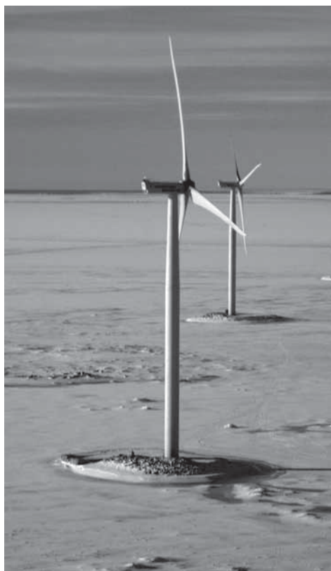
Figure 4 New semi-offshore wind farm (ten 3-MW WinWinD turbines) installed in Kemi Ajos. (Photo: Eero Kokkonen, PVOI).
