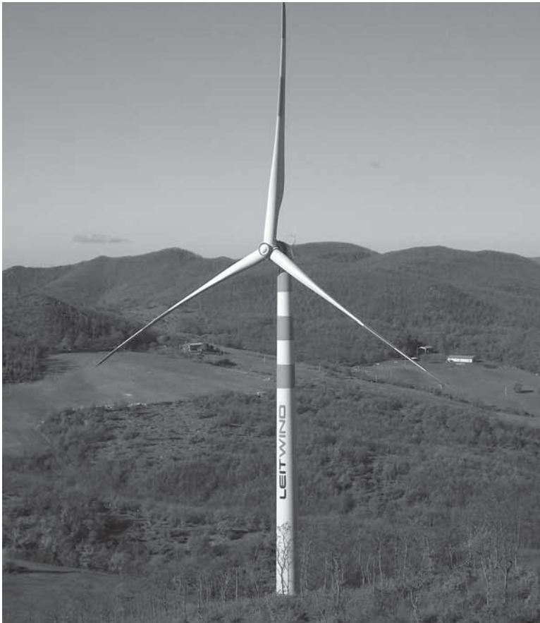
Figure 7 Leitwind LTW 77 1.5-MW turbines installed in Tuscany (courtesy of Leitwind).
