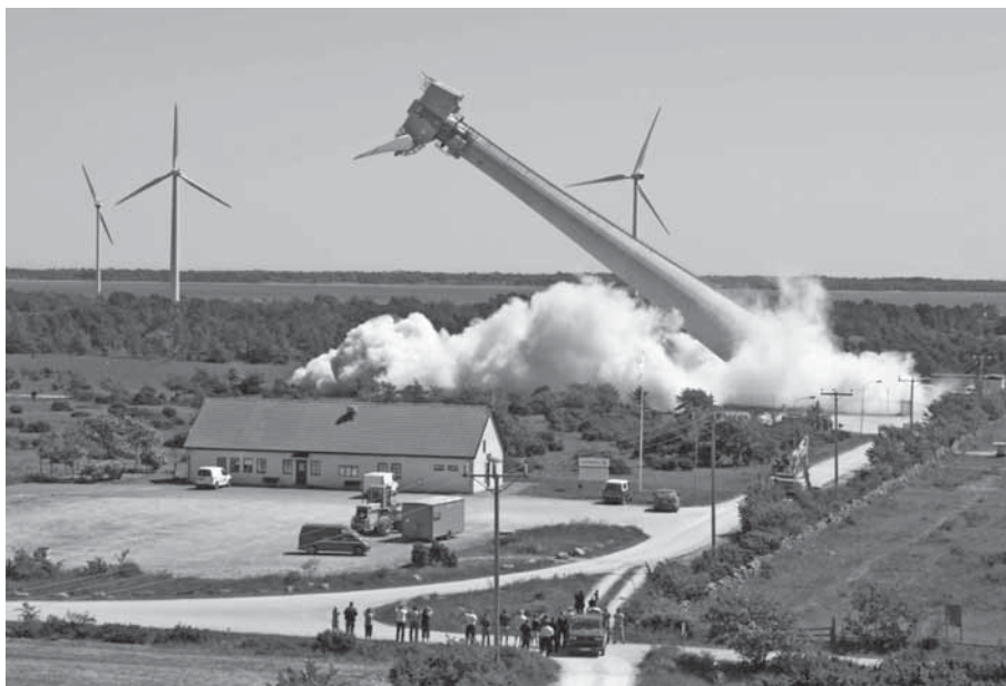
Figure 3 The decommissioning of wind power aggregate Näsudden II.
