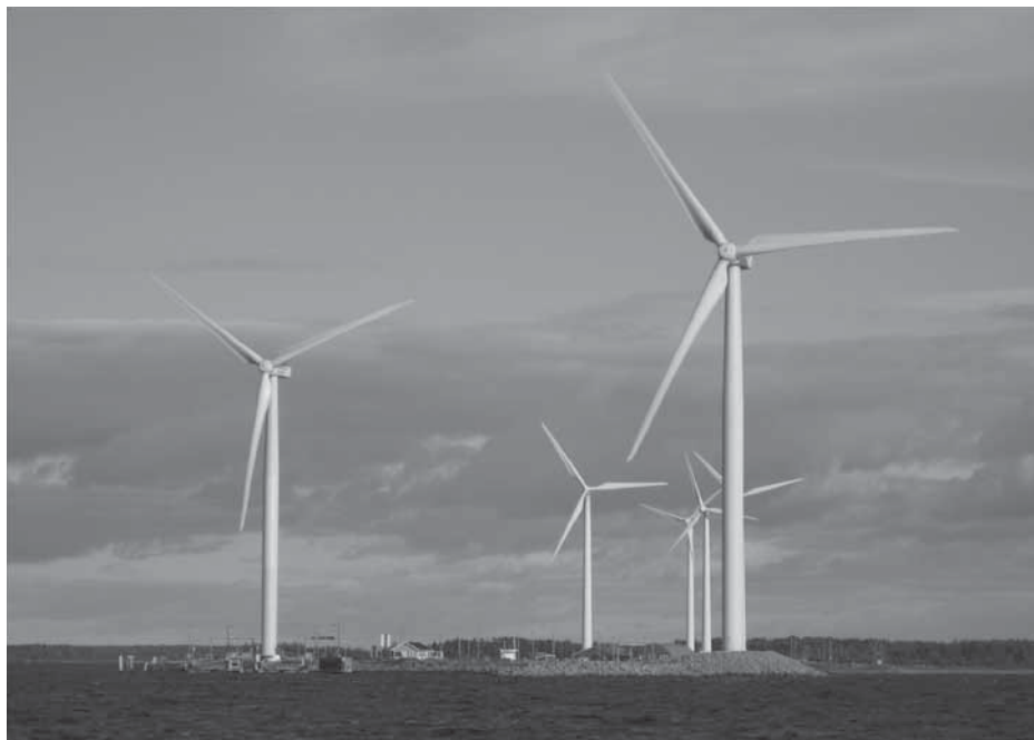
Figure 2 Oulunsalo saw two new 3-MW WinWinD turbines added to the existing wind park in 2008 (three 1-MW WinWinD turbines; one 1.3-MW Nordex turbine). (Photo: WinWinD).
