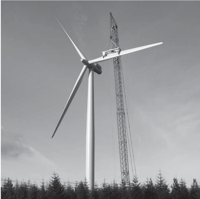
Figure 1 The final blade is fitted to the first turbine on Whitelee wind farm. Image courtesy of Scottish Power Renewables.
