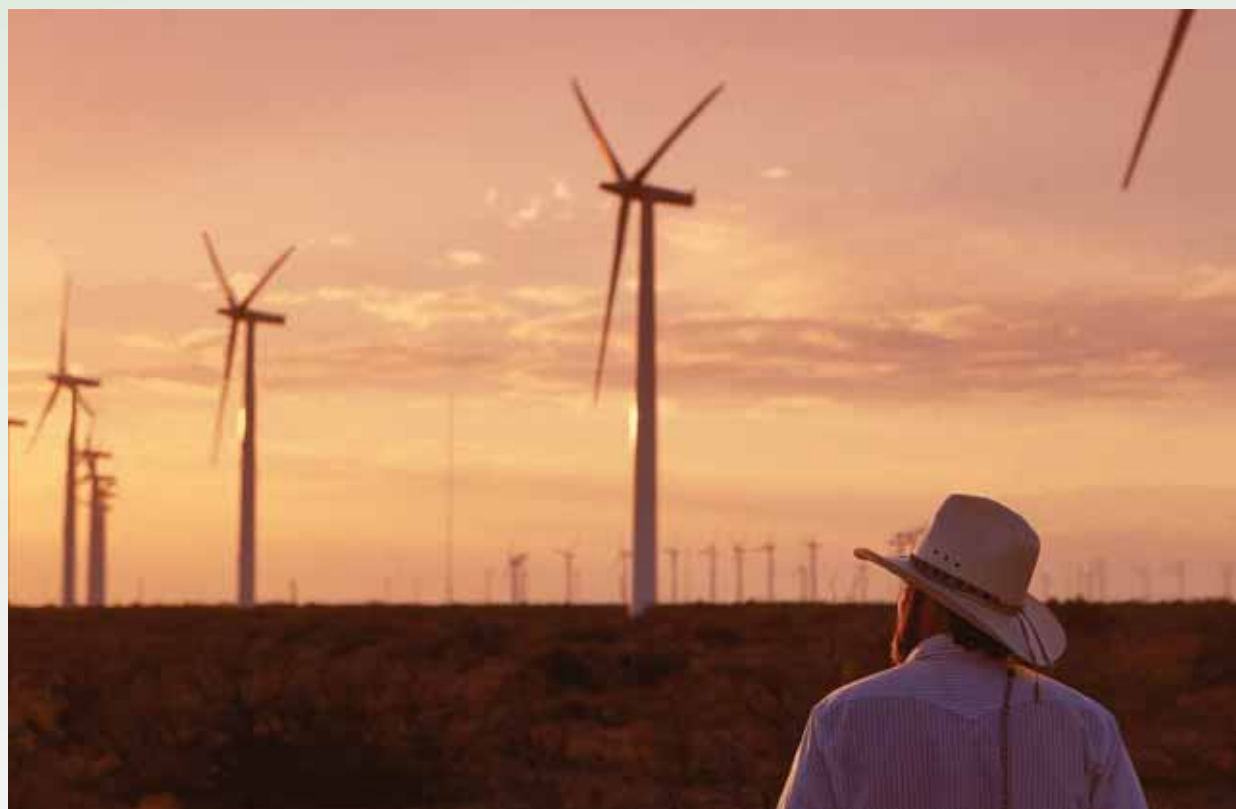
Figure 1 The 781.5-MW Roscoe Wind Farm, in Texas provides 70 full-time jobs for plant operations
