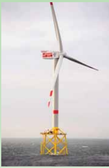
Figure 3 Repower 5M on a jacket foundation at alpha ventus ©alpha ventus picture library
