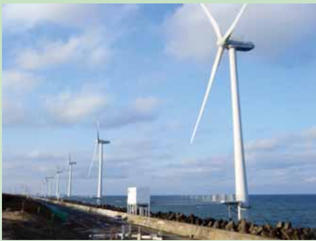
Figure 3 The 14-MW offshore wind plant in Kamisu, Ibaraki.
