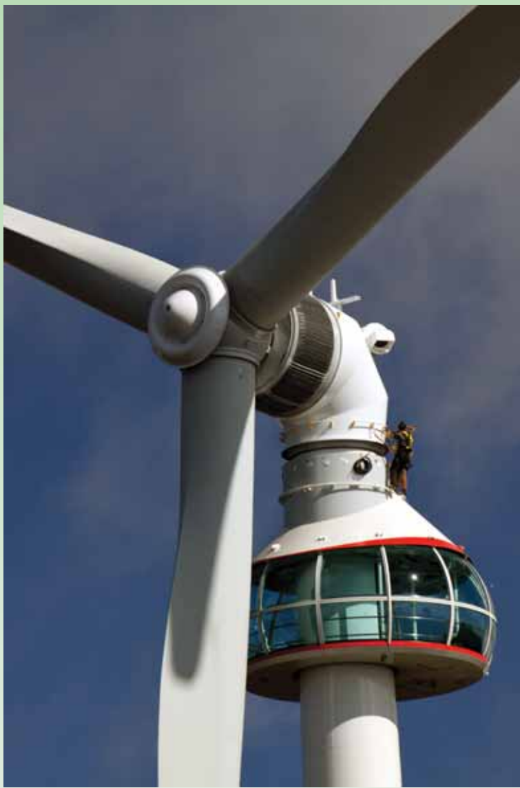
Figure 4 Leitwind 1.5-MW LTW77 wind turbine with panoramic platform installed on Grouse Mountain near Vancouver, Canada (courtesy of Leitwind)
