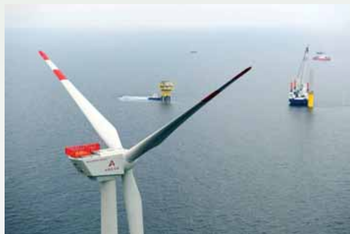
Figure 2 The first offshore wind turbine of alpha ventus with the transformer station in the background. ©alpha ventus picture library
