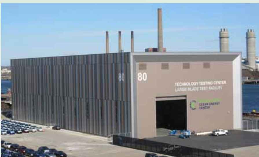
Figure 3 The new DOE/NREL/MassCEC large blade test facility, the Wind Technology Testing Center (WTTTC), under construction in Boston, Massachusetts
