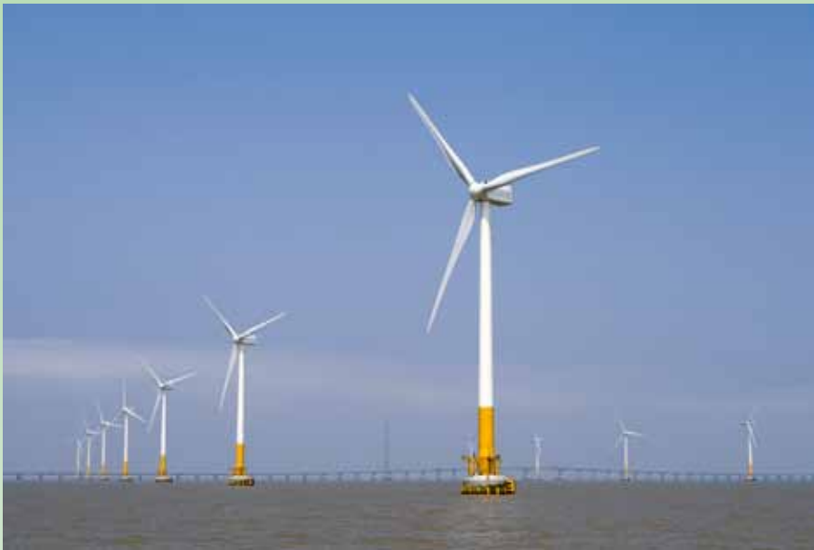
Figure 3 The first offshore wind farm in China began operation in 2010. It is 102 MW and located near Shanghai Donghai Bridge.
