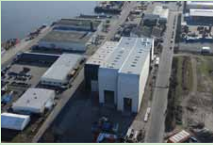
Figure 4 The 90 m test rig for rotor blades next to the 70 m test rig at IWES
