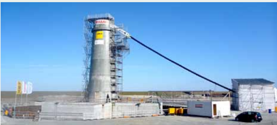
Figure 5 The gravity test foundation of Ed. Züblin AG in Cuxhaven
