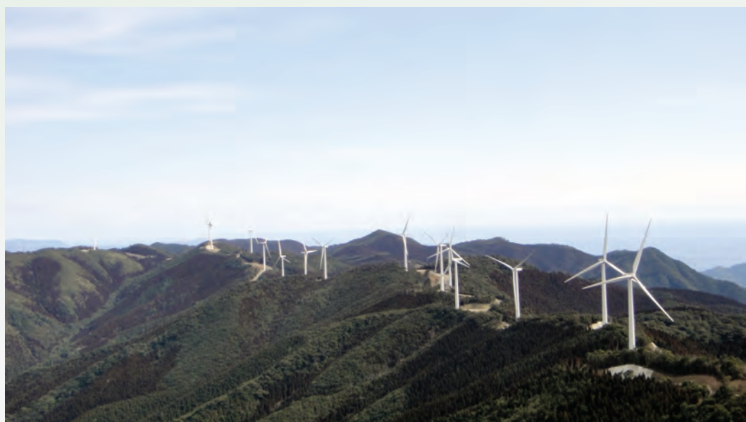
Figure 2. Kunimiyama windfarm, with 15 of JSW's 2-MW turbines. Operation began in March 2011. (Source: Eurus Energy Holdings Co.)
