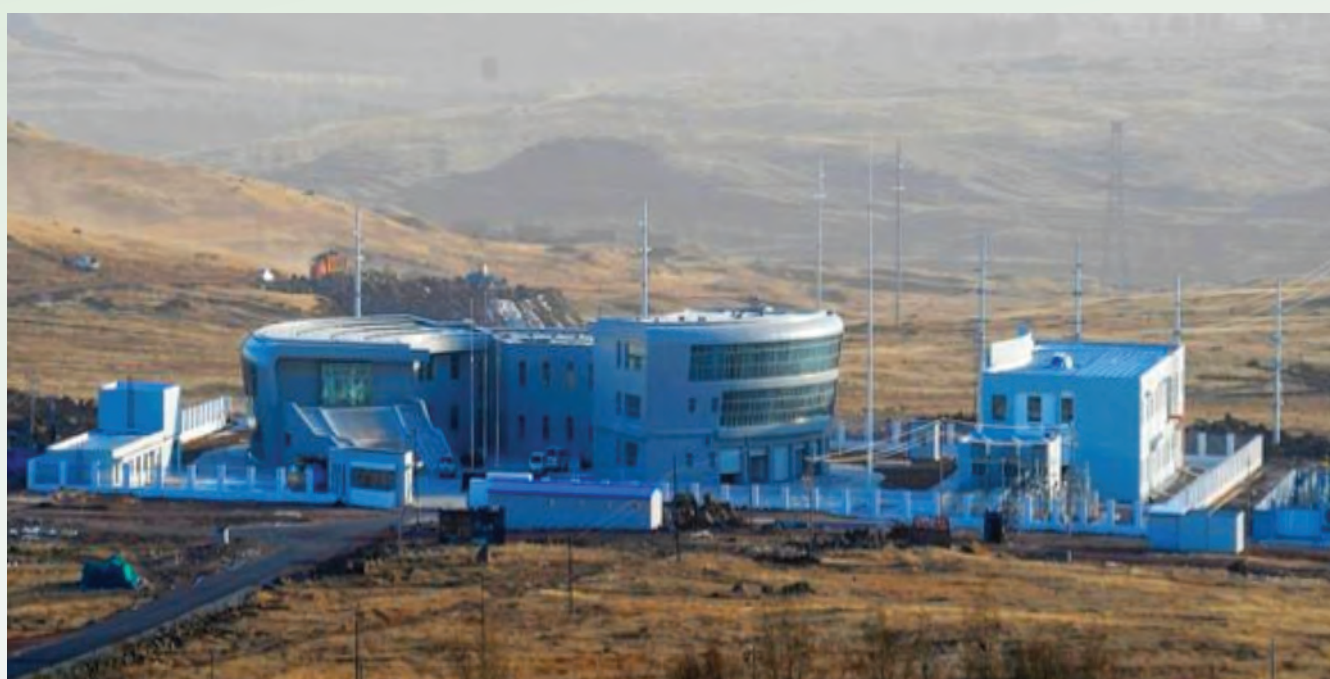
Figure 4. National Wind Power Integration Research and Test Center
