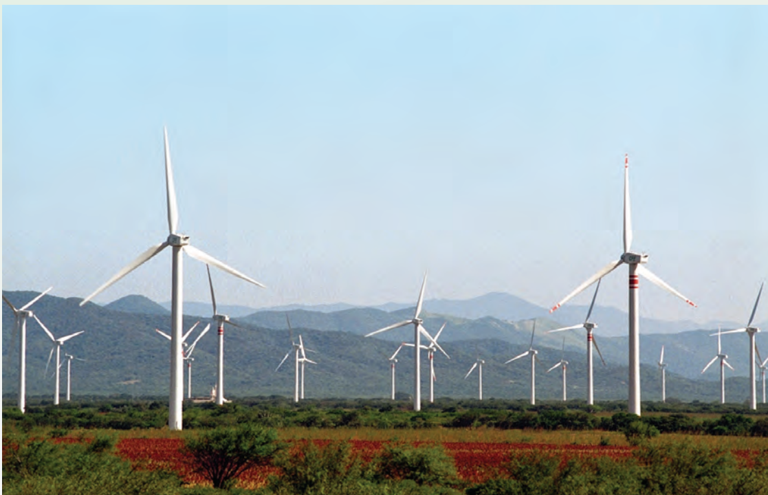
Figure 2. La Venta II 83.3-MW wind farm in the Isthmus of Tehuantepec, México
