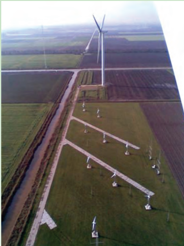
Figure 3. The nine small wind turbines at the ECN Wieringermeer test field are used to measure and model the wake in a wind farm (Photo: ECN)
