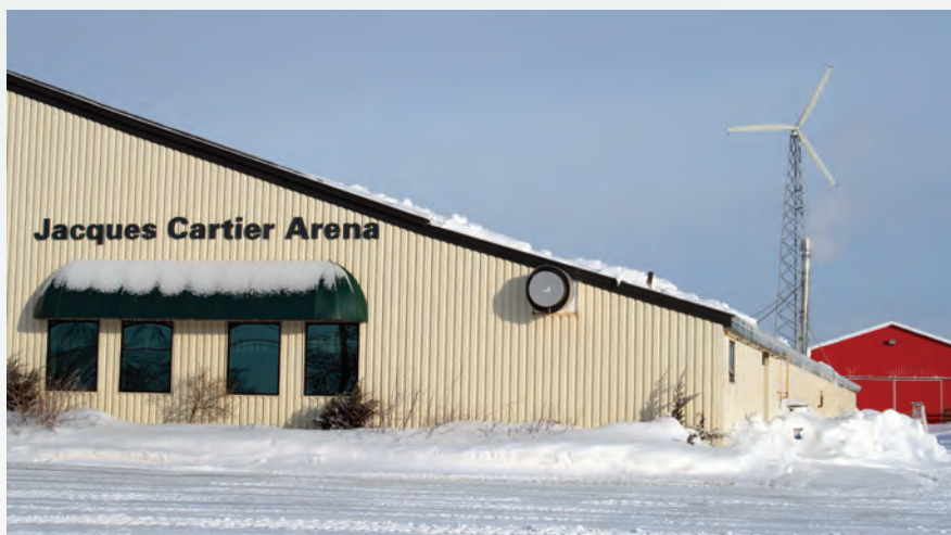
Figure 1. Wind turbine powering Jacques Cartier Arena in PEI Source: WEICan
