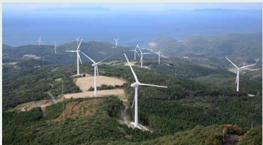
Figure 2. Kushikino-Reimei wind power plant has ten 2-MW Hitachi HTW 2.0-80 turbines and began operation in December 2012. Source: Kyudenko Co., Inc.
