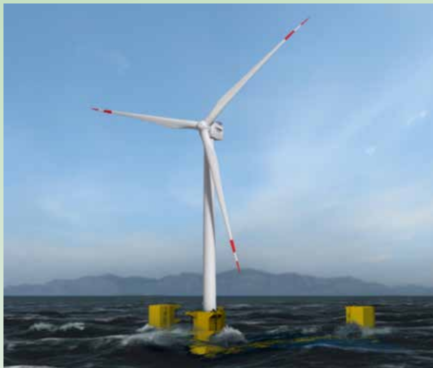
Figure 4 Conceptual CG image of offshore floating offshore wind farm in the METI Floating Offshore Wind Farm Demonstration Project (Source: Fukushima FORWARD).
