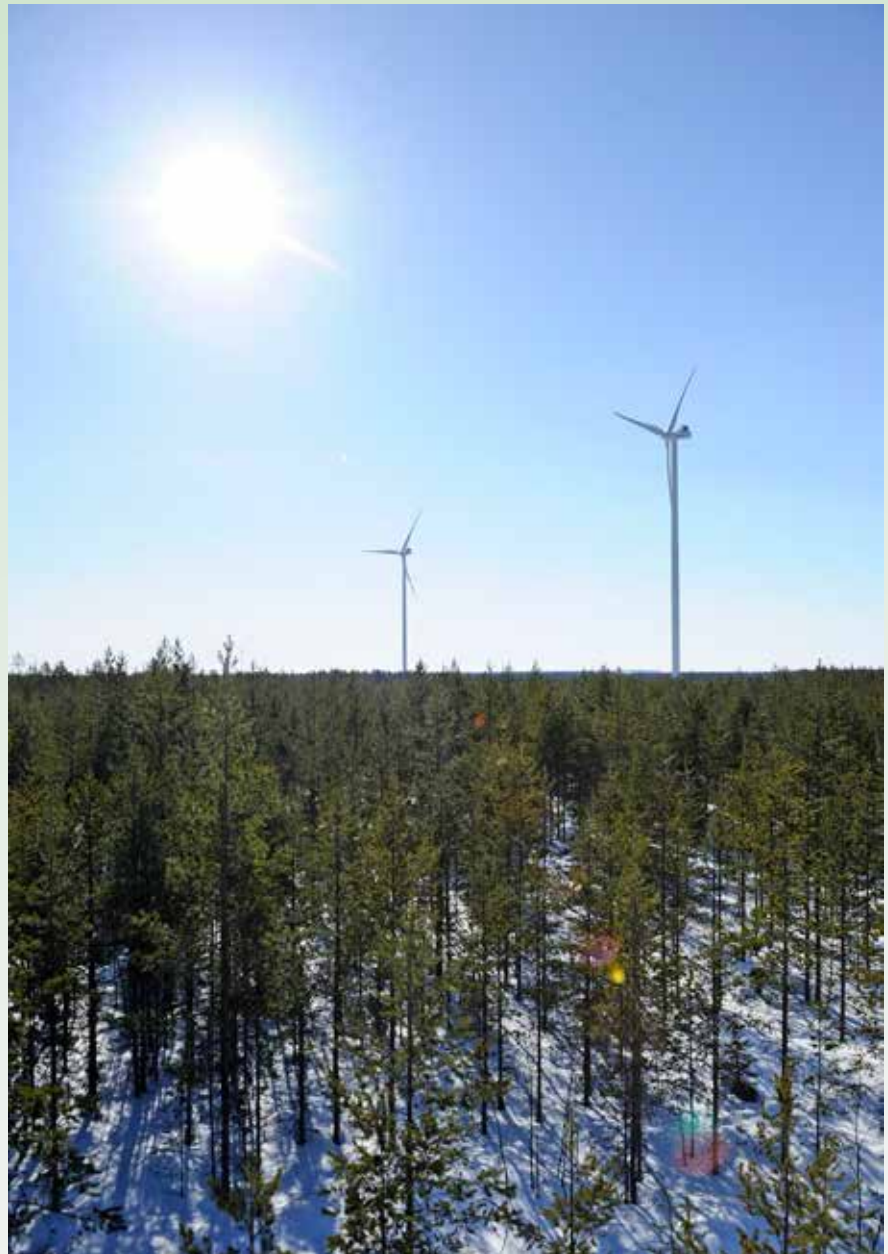
Figure 4. Olhava wind power plant. (Source: Tuuliwatti)
