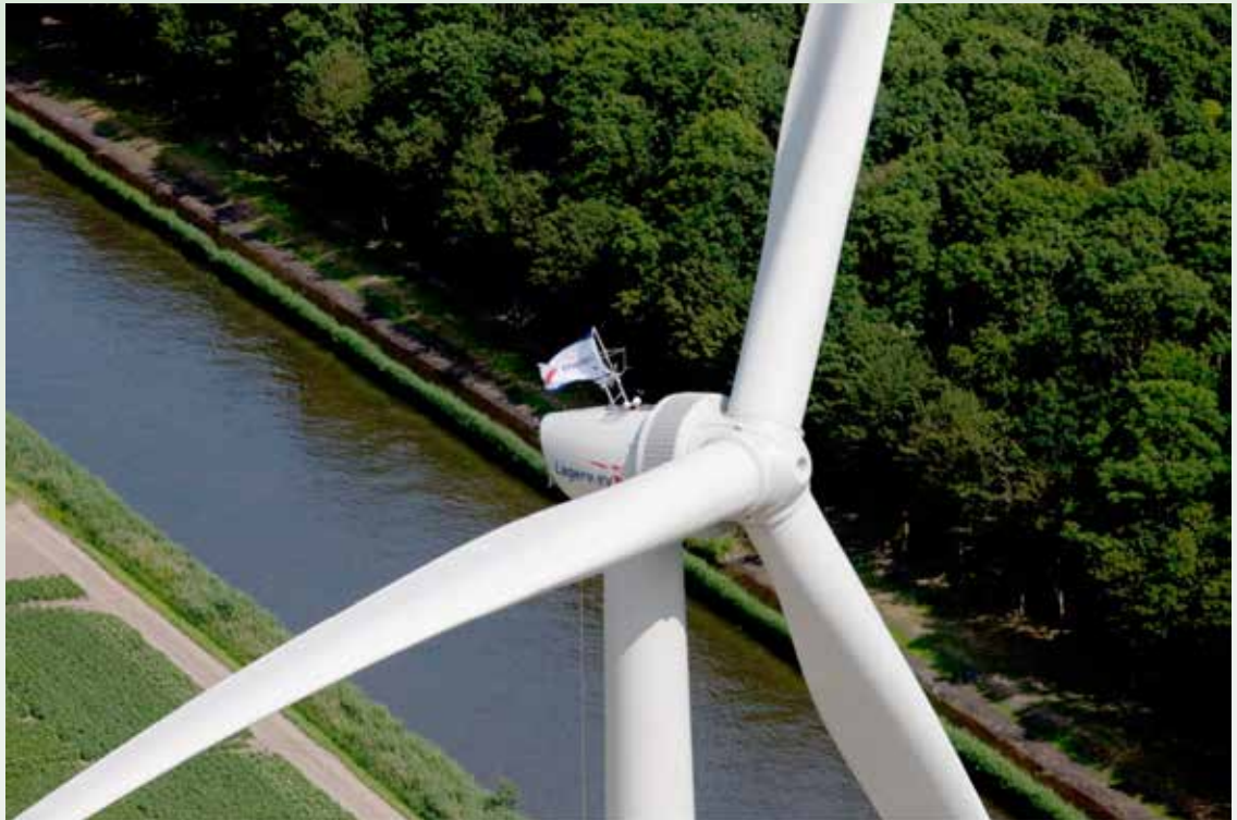
Figure 1. The first new L93 Lagerweij 2.6-MW turbine becomes operational
