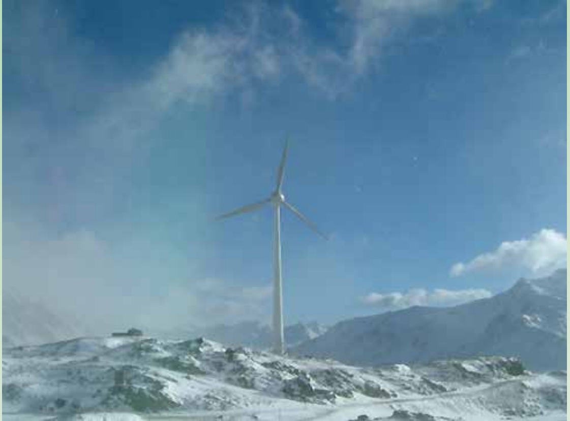
Figure 1. Wind turbine in Gütsch (Source: Suisse Eole)
