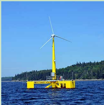
Figure 1. The University of Maine's 1:8th-scale offshore wind demonstration project (Photo by University of Maine)
