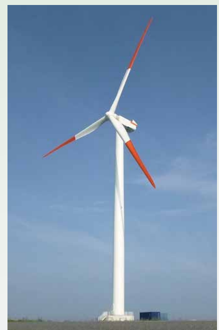
Figure 3. The new JSW 2.7-MW wind turbine "J100-2.7"
