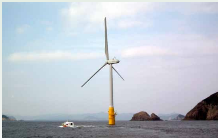
Figure 5. Hitachi 2-MW wind turbine with spar type floater in the MOE floating offshore wind turbine demonstration project (Source: MOE)
