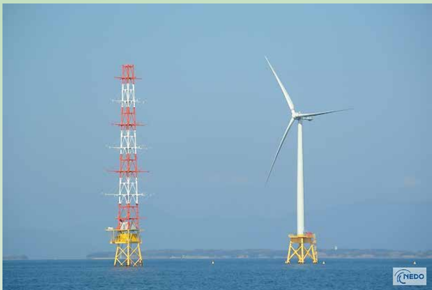
Figure 4. JSW 2-MW wind turbine and offshore measurement platform on the jacket and gravity hybrid foundation in Hibikinada offshore wind power demonstration project (Source: NEDO)
