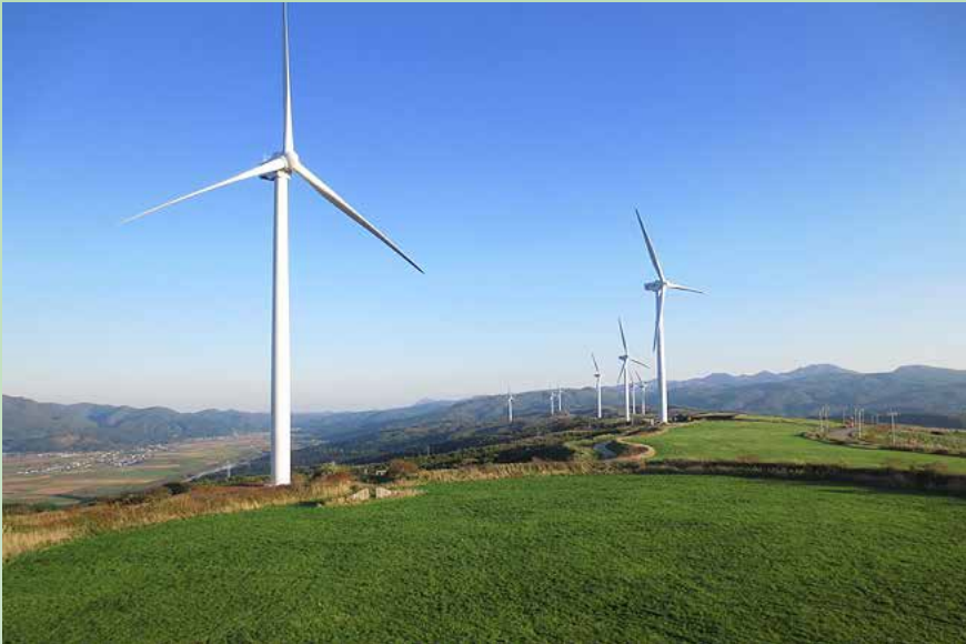
Figure 2. Kaminokuni Wind Farm in Hokkaido prefecture—12 MHI 2.3-MW turbines with a total capacity of 28 MW (Source: Electric Power Development Co., Ltd. (J-POWER))
