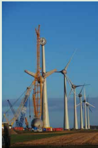
Figure 5. Enercon E-126 turbines being assembled along the dike at Noordoostpolder wind farm
