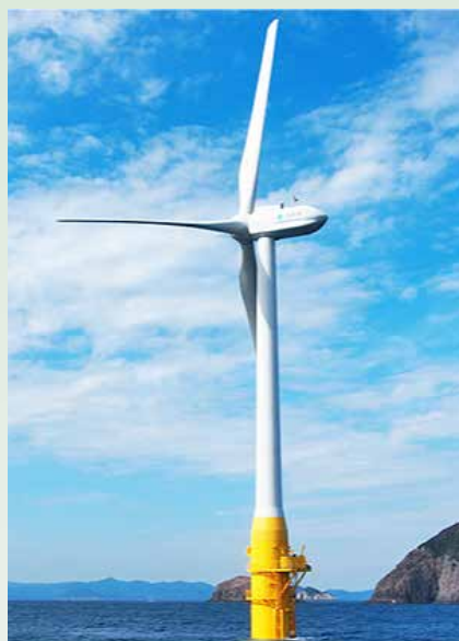
Figure 4. Hitachi 2-MW wind turbine with spar type floater in the MOE floating offshore wind turbine demonstration project (Source: GOTO-FOWA PJ)
