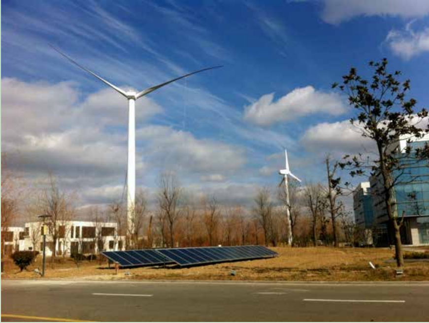
Figure 3. Wind-photovoltaics-storage intelligent micro-grid application project in Yancheng
