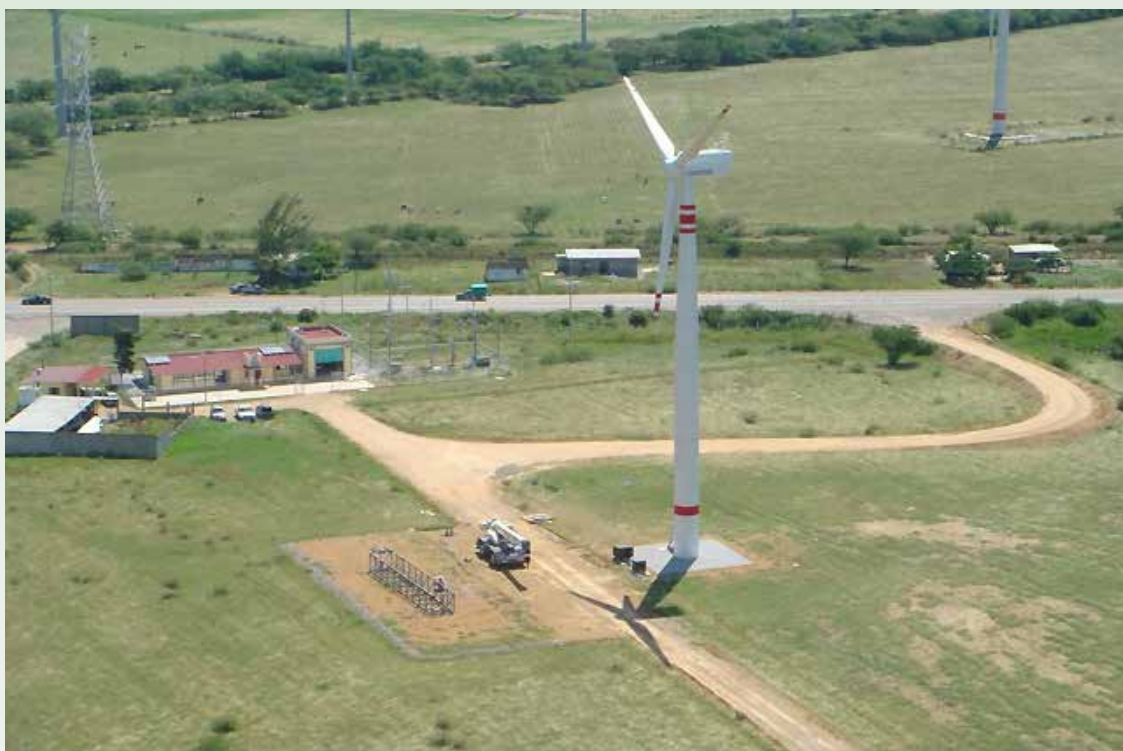
Figure 1. The Wind Turbine Test Center operated by the Instituto de Investigaciones Eléctricas
