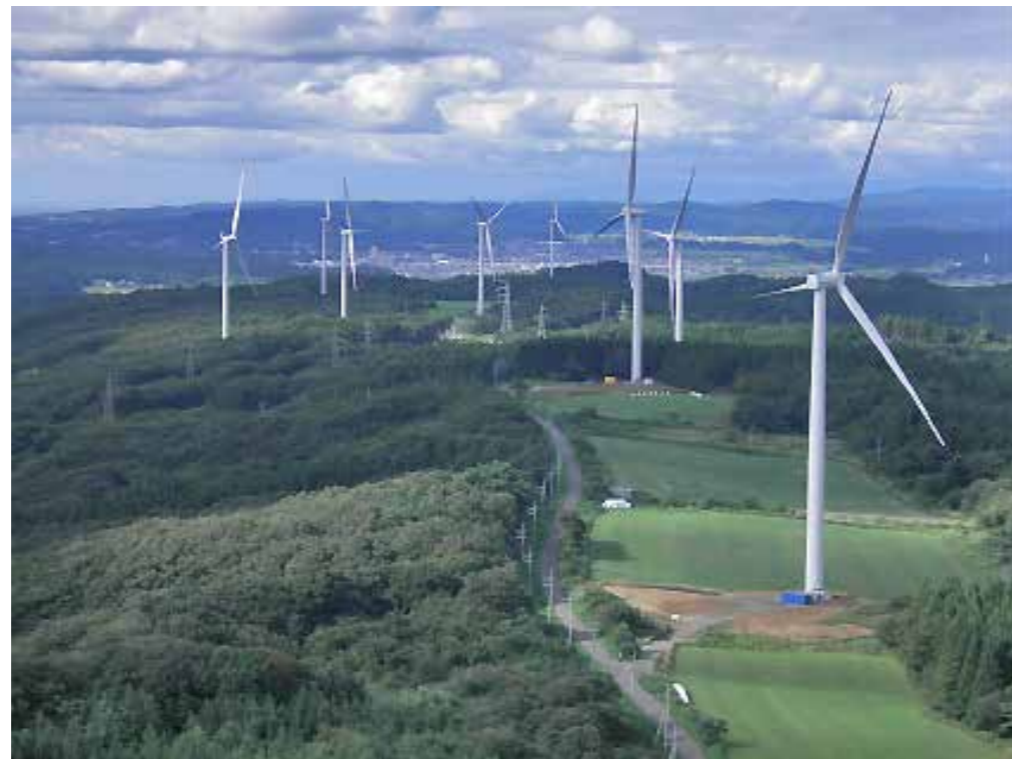
Figure 2. Eurus Yurikogen Wind Farm in Akita prefecture: 17 Siemens 3-MW turbines with total capacity of 51 MW (Source: Eurus Energy Holdings Corporation)
