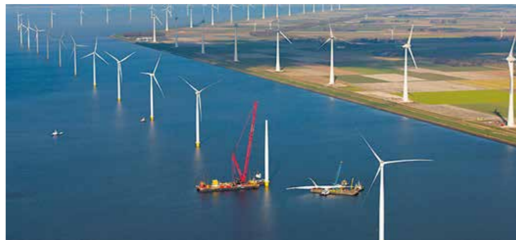
Figure 1. The last wind turbine being placed in Lake IJsselmeer at the Westermeerwind/Noordoostpolder wind farm
