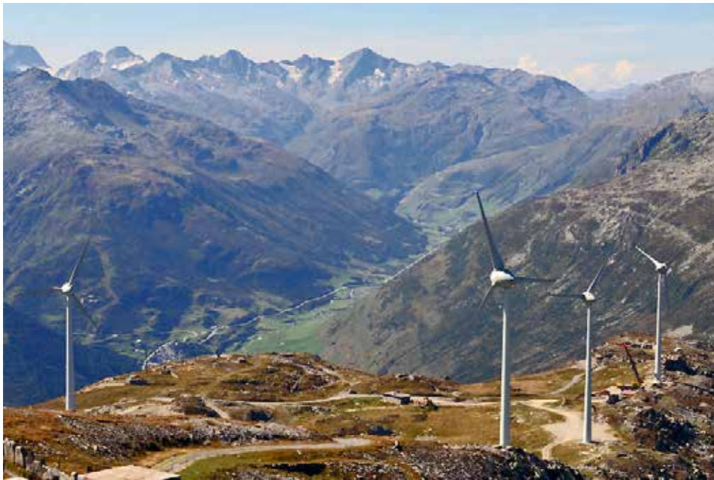
Wind farm in Gütsch (Photo credit: ©SwissEole)
