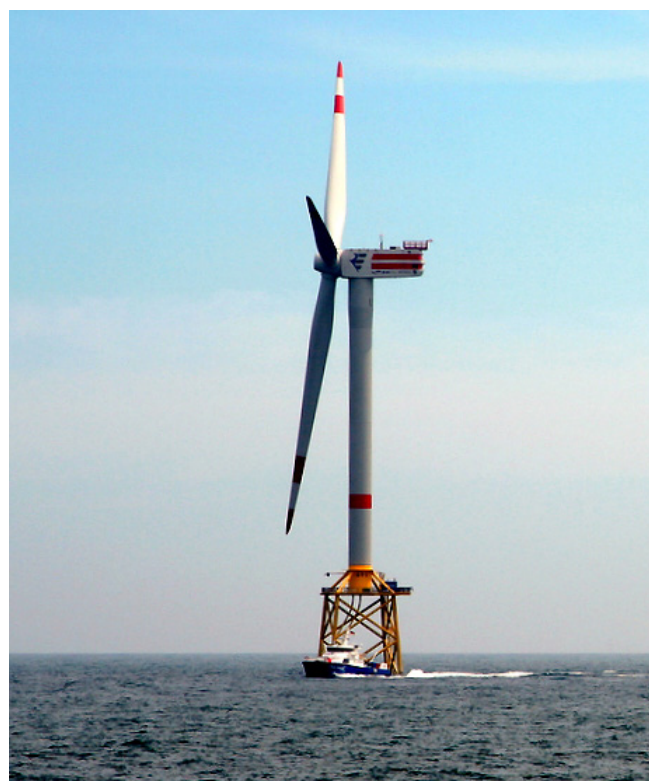
Figure 12. Offshore wind system examined in IEA Wind TCP Task 30 OC5 Phase III: Jacket – Open Ocean Test (Photo Credit: Gary Norton, NREL)
