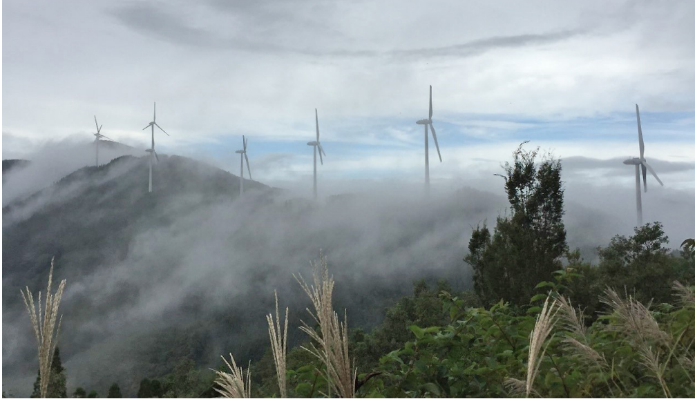
Figure 2. The JRE Nakakyushu-Onitayama Wind Farm in Miyazaki prefecture (Hitachi 2-MW 8 turbines with total capacity of 16 MW) began operation in September 2016 (Source: Japan Renewable Energy Corporation, JRE)
