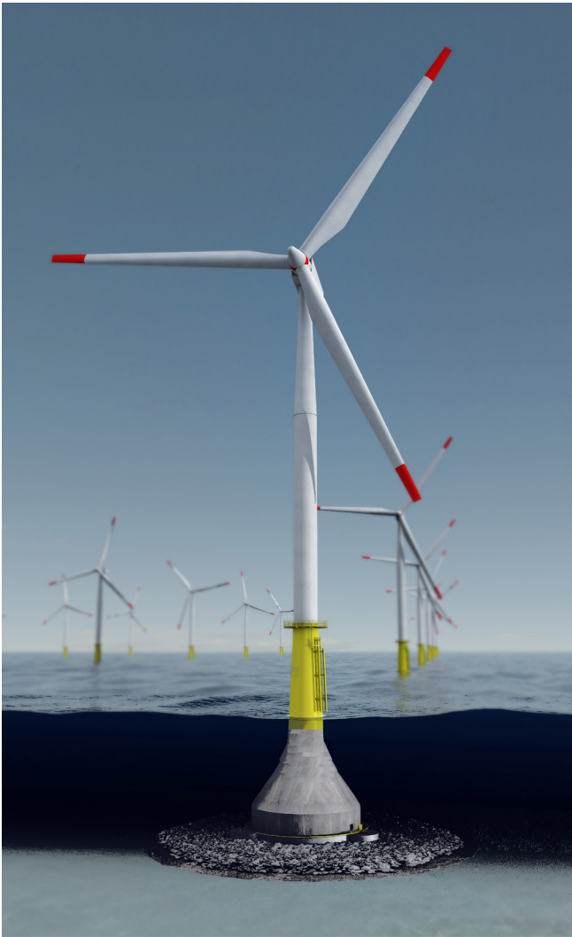
Figure 3. With Seatower's Crane-free Gravity® foundation, seawater flows into a hollow foundation at the base of a turbine. This fixes the structure to the seabed, speeding up installation time and minimizing risk. (Photo credit: Seatower)
