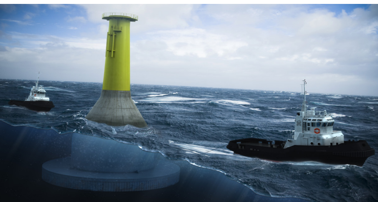
Figure 2. Seatower has developed a gravity based foundation with crane free installation. A pilot foundation supports a met mast at the planned Fécamp wind park in French waters. (Photo credit: Seatower)
