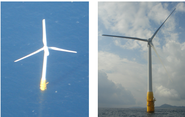
Figure 3. Hitachi 2-MW floating offshore wind turbine at Fukuejima in the Nagasaki prefecture (Photo credit: Ueda, Y., JWPA)
