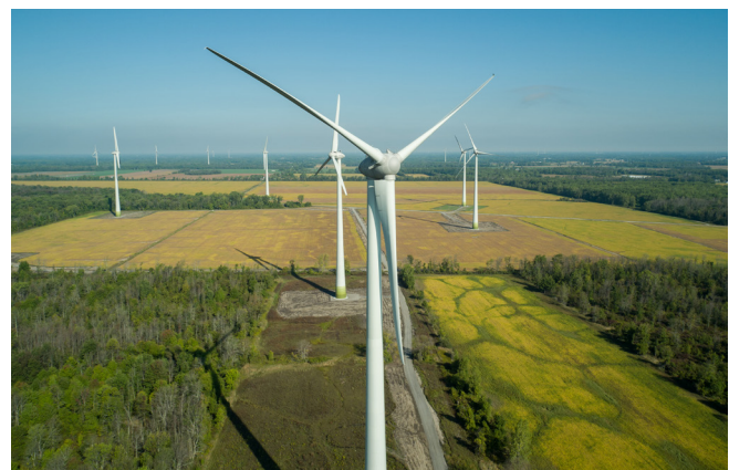
Figure1. Enercon E-101 3 MW turbines in the Niagara Region Wind Farm, Ontario, Canada (Source: © Enercon Canada Inc.)
