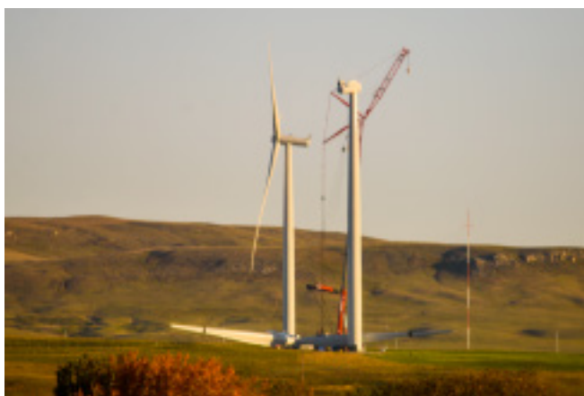
Figure 2. Turbine under construction, Piikani Nation, Alberta, Canada (Photo credit Jaq Murillo)
