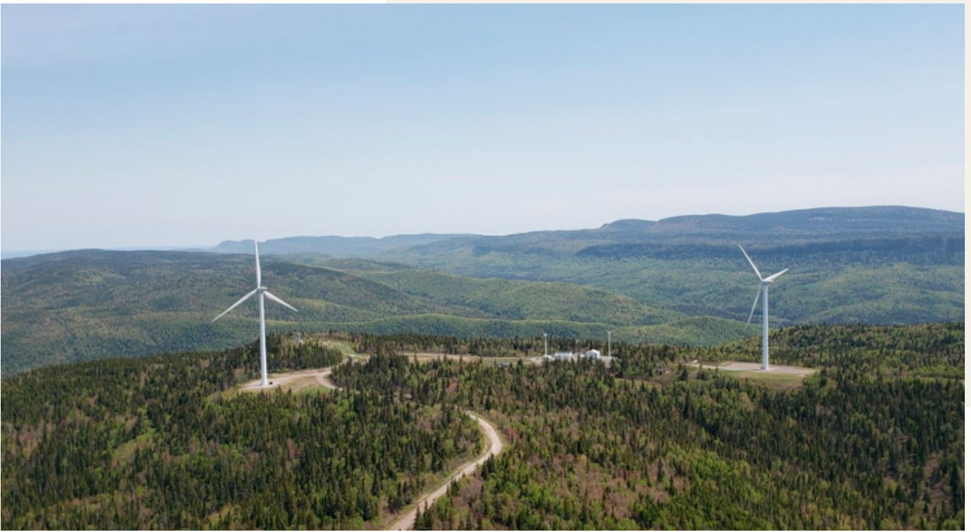
Nergica research site, Quebec, 2 Senvion MM92 CCV, 4.1 MW installed capacity, plus a 230 kW Diesel, Wind, and Solar microgrid. Source: Nergica.
