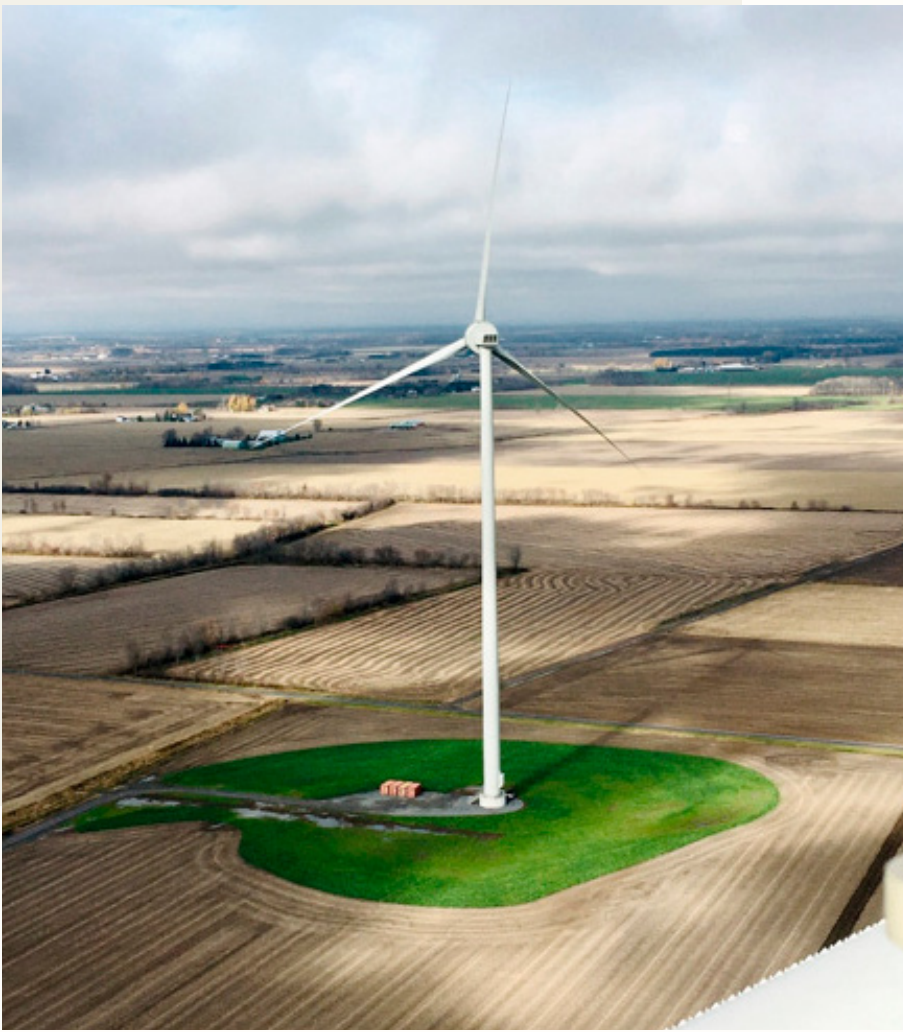
Picture: 100 MW wind farm in Nation Rise, ON. Wind Turbine Model E-138 EP3, Source: ENERCON Canada Inc.
