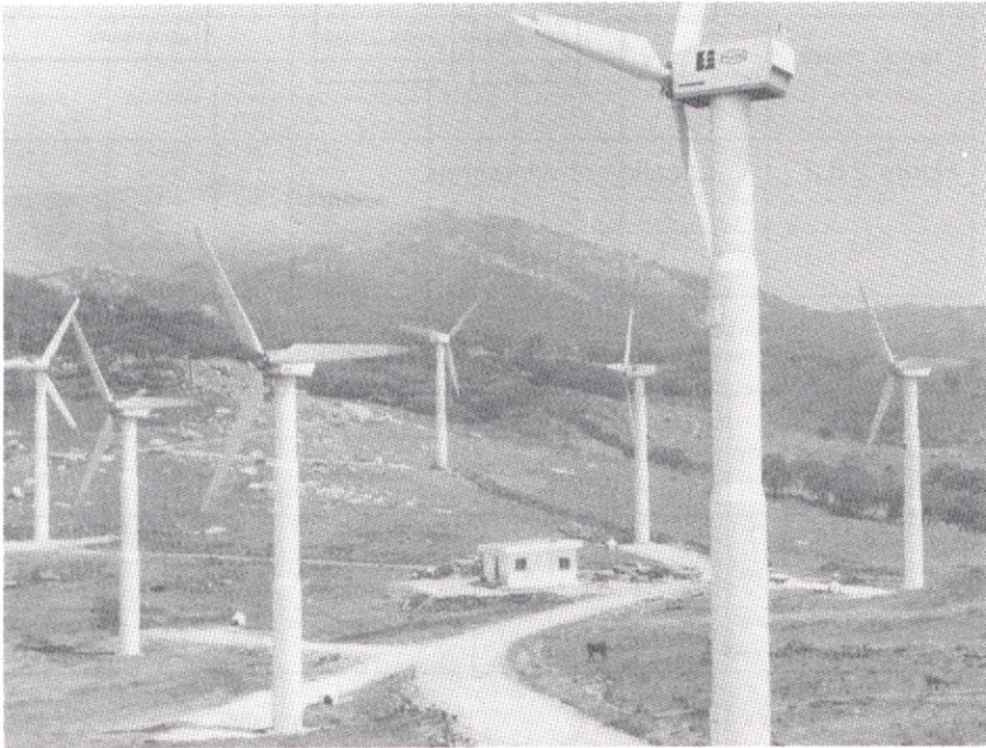
Figure 2.8.4 The Monte Ahumada windfarm at Tarifa
