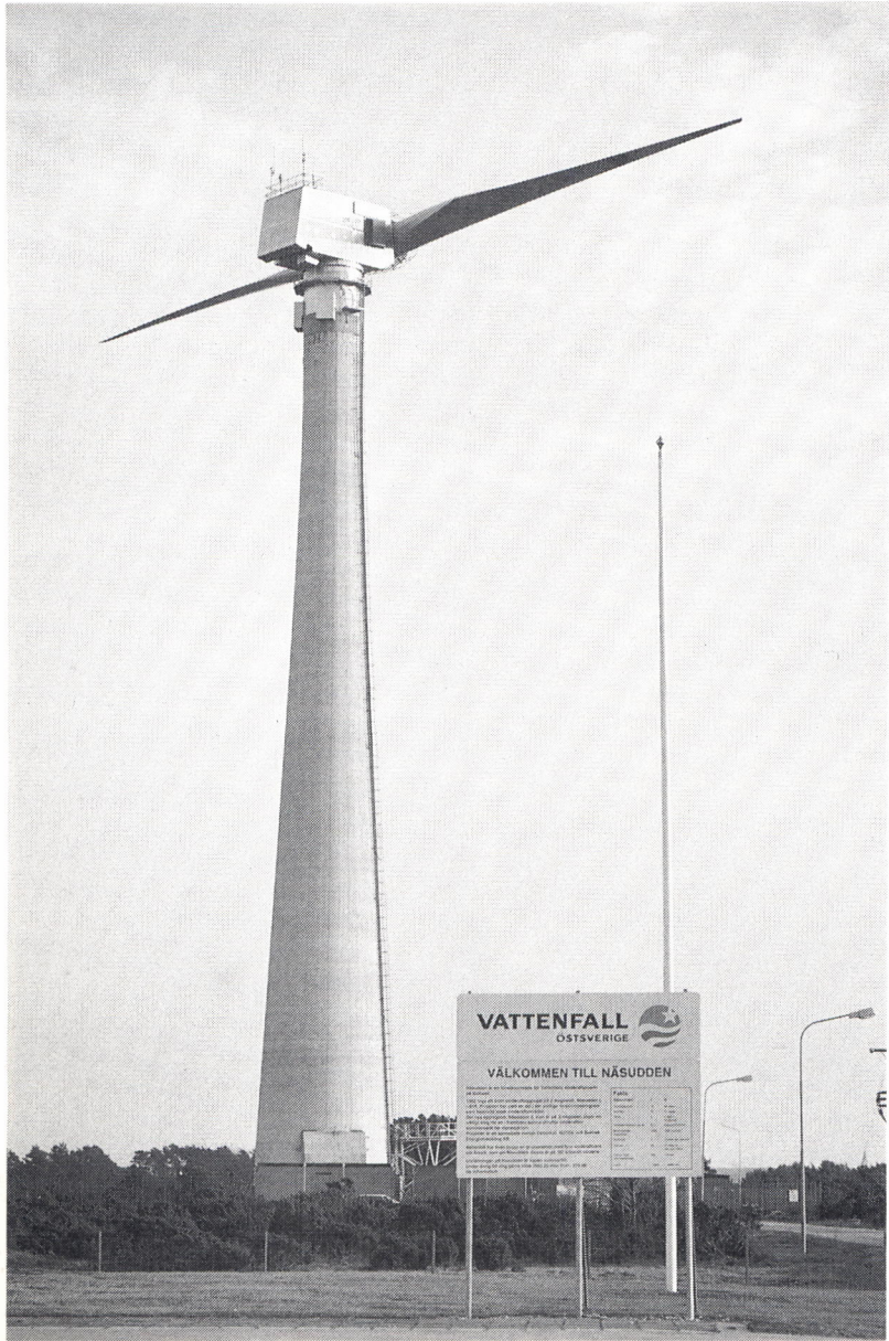
Figure 2.9.1 The 3 MW Näsudden II. Rotor diameter 80 m
