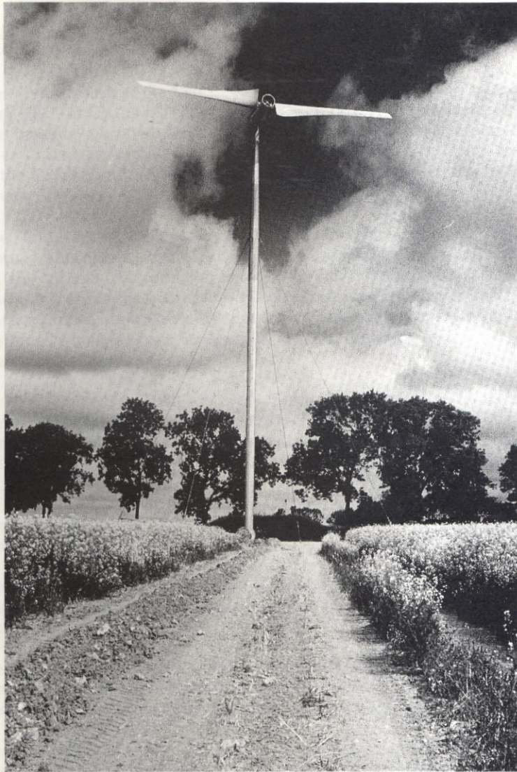
Figure 2.11.3 The North Wind 250 wind turbine
