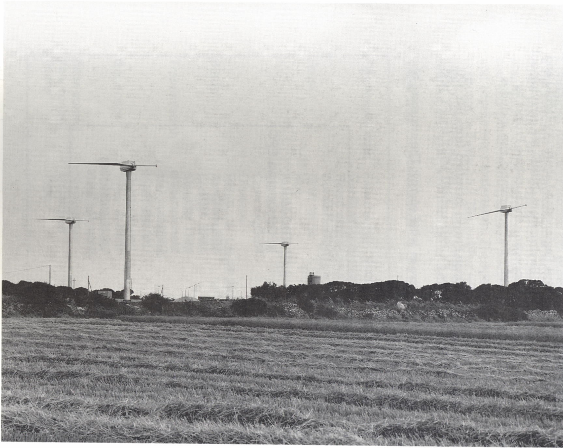
Figure 2.4.5 The wind farm set up in 1993 in Northern Sardinia for "Consorzio di Bonifica di Nurra": view of the Ottava plant with four Riva Calzoni M30-A wind turbines
