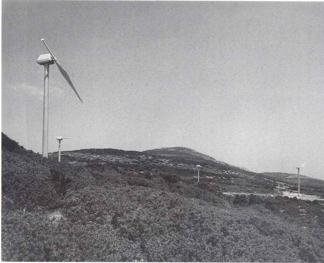
Figure 2.4.4 The wind farm set up in 1933 in Northern Sardinia for "Consorzio di Benifica di Nurra": view of the Campanedda plant with four Riva Calzoni M30-A wind turbines
