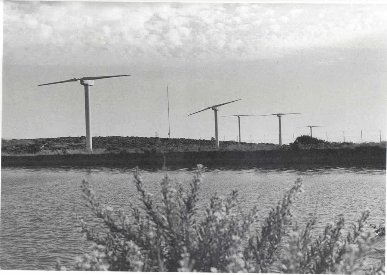
Figure 2.4.1 The windfarm set up in 1933 in Northern Sardinia for "Consorzio di Bonifica di Nurra: view of the Monte Uccari plant with five WEST Medit 320 machines
