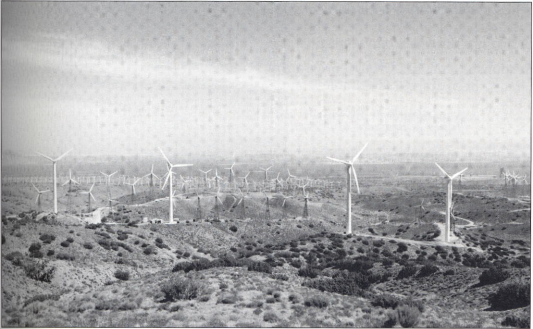
Figure 12. Example of industrial trade. 4 Tacke TW 600 at Tehachapi, California, 1994. The 500 kW prototype was supported by BMBF (see Figure 1)
