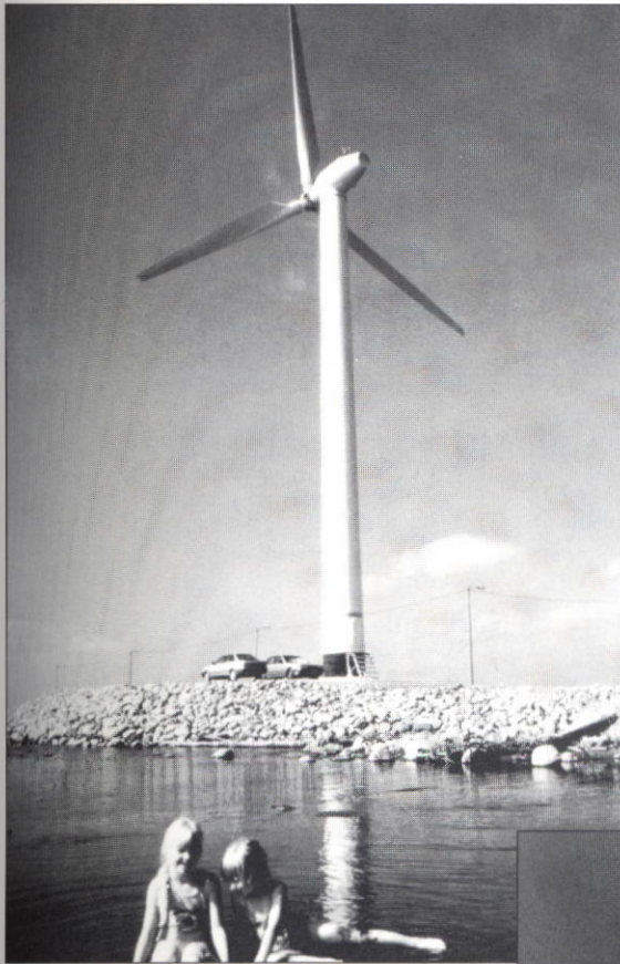
Figure 2. Nordtank 300 kW turbine in Siikajoki, Finland, close to a small fishing harbor (Foto Revon Sähkö Oy)
