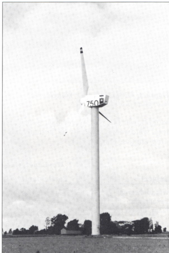
Figure 2. HSW 750. Prototype at the test site Kaiser-Wilhelm-Koog. HSW 1000, summer 1995. Rated power: 1 MW. Rotor \varnothing : 54 m, pitch. Hub high: 55 m. Steel tower. Nacelle with rotor: 73.000 kg
