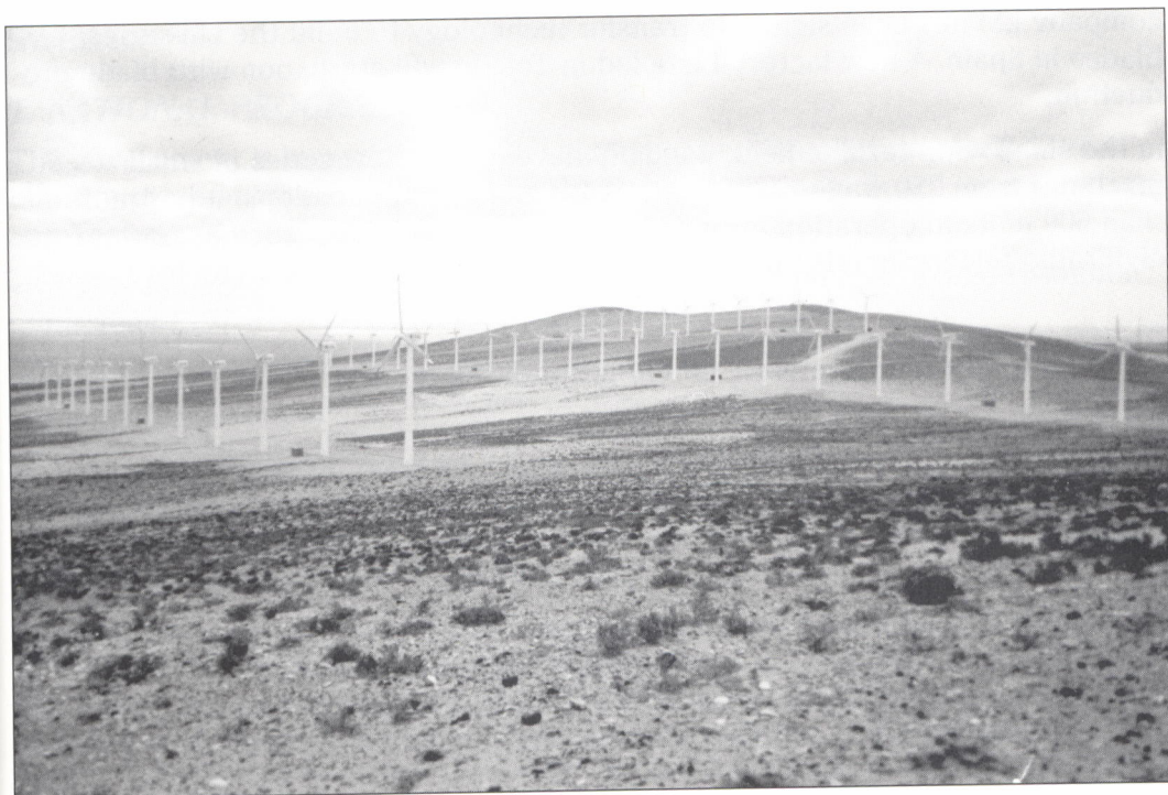
Figure 7. Canada del Rio Wind Farm 10.8 MW
