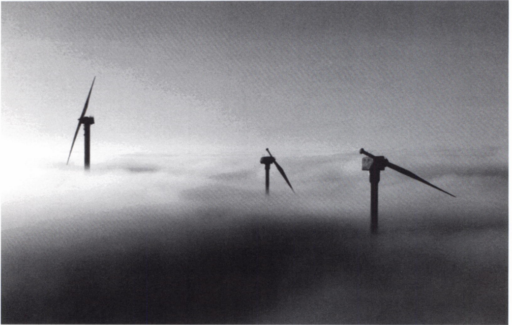
Figure 3. AEOLUS II (left) near Wilhelmshaven, seen from the nacelle of one of the three 640 kW MONOPTEROS single-bladed WECs.
