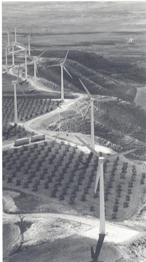
Figure 3. La Muela wind power plant (Ebro Valley) 330 kW wind turbines.
