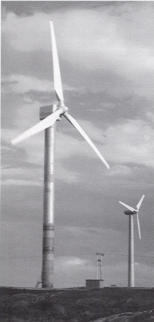
Figure 1. Wind turbines at the test site Frøya. The 55 kW turbine in the background is part of the wind/diesel system.
