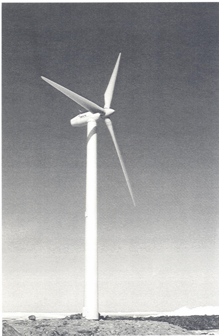
Figure 3. The first 500 kW turbine in Finland was installed in April 1995 in Hailuoto close to two 300 kW turbines.
