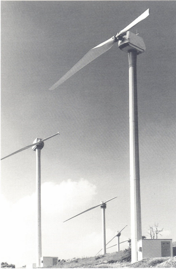
Figure 1. Partial view of the 3.5 MW wind power plant built by Riva Calzoni at Casone Romano (southern Italy) with ten units supplied by the same firm.
