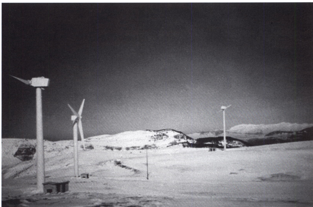
Figure 4. View of ENEL's Acqua Spruzza test site in the Apennines (1,360 m above sea level) after a snowfall, with three of the eight machines.
