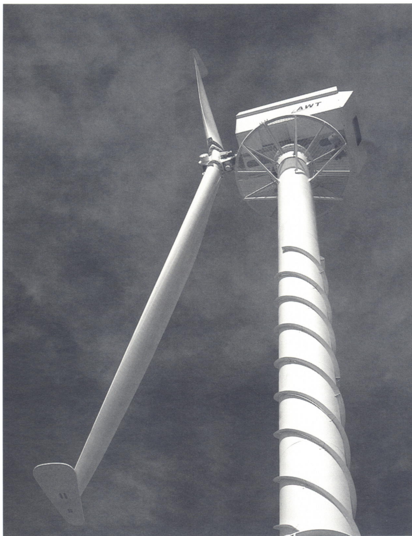
Figure 2. AWT-26 prototype, 275 kW, 26 m rotor diameter advanced turbine operating at the National Wind Technology Center near Golden, Colorado.
