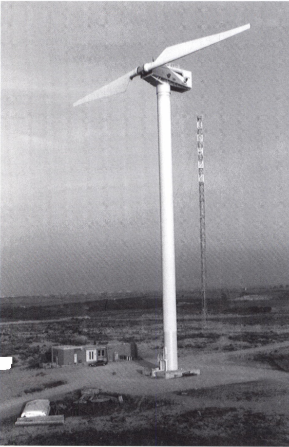
Figure 2. The 1.5 MW GAMMA 60 prototype at Alta Nurra. Fine-tuning of the GAMMA project is under way, with a possibility of manufacturing two pre-series units.
