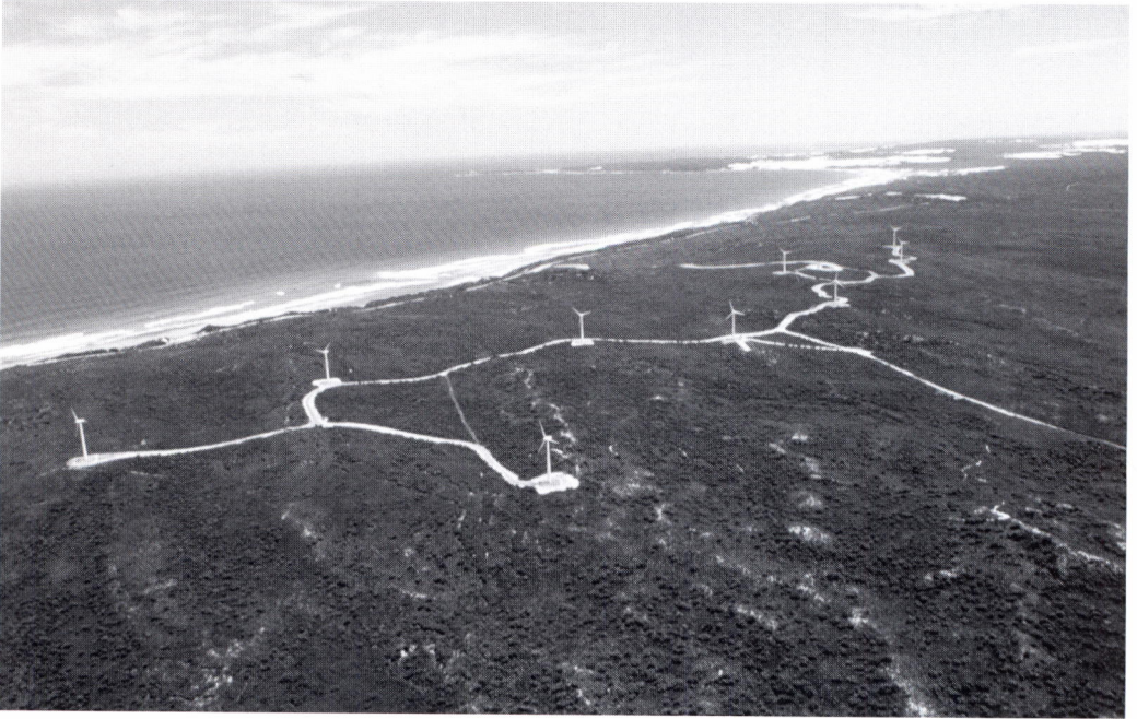
Figure 1. View of the 2 MW Ten Mile Lagoon wind power plant (nine 225 kW Vestas machines).
