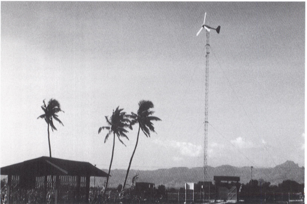
Figure 4. BWC 1500-PD, 1.5 kW, 3 m rotor diameter, Bergey Windpower turbine in the Indonesian village of Oesao, used for wind-electric water pumping that irrigates four hectares of vegetable farms.
