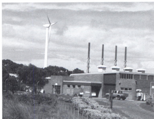
Figure 8.4 Huxley Hill wind-diesel installation, Australia
