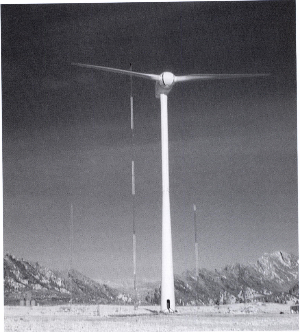
Figure 22.8 This 250-kW proof-of-concept turbine has hinged rotor blades
