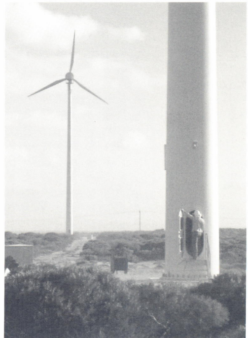
Figure 8.3 Showcase installation at Denham, Australia (0.69MW)
