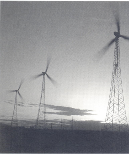
Figure 22.1 This 193-MW wind power plant at Storm Lake, Iowa uses Zond Energy Systems 750-kW turbines
