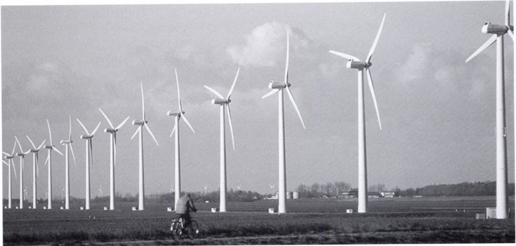
Figure 17.3 Wind farm of 11.4 MW consisting of 19 NEG-Micon 600-kW, 48m diameter turbines in typical farming country. This is the largest wind farm built in 1999 on the land of farmers. It is owned and exploited by a private company in which five or six farmers hold the shares.
