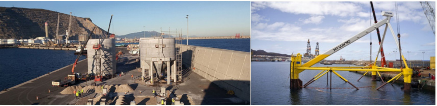
Figure 3: Left: DemoSATH floating offshore wind platform (Bilbao Port, Spain). 2 MW Full scale prototypes. (Credit: SAITEC) Right: Pivotbuoy. Floating offshore wind platform 1:3 partial scale prototype (Las Palmas Port, Spain). (Credit: X1 Wind).
