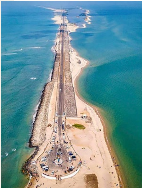
Source: Dhanuskodi (Planned for Offshore Test Facility)
