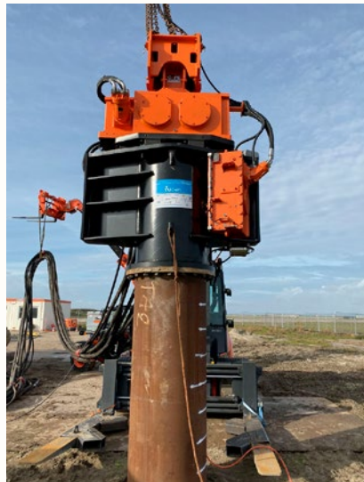
Picture 3. Gentle Driving of Piles (GROW Offshore Wind)
