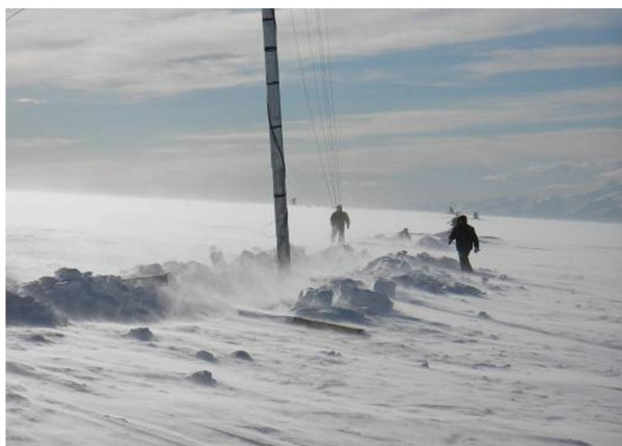
Figure 4-4 Winter meteorological tower installation in Alaska. Photo: Doug Vought, USA
