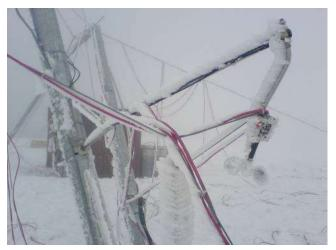
Figure 4-1: A collapsed meteorological tower, likely due to heavy icing.
