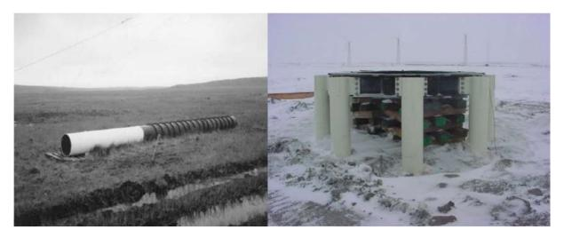
Figure 5-2: Freeze-back pylons used for turbine (and other) foundations in permafrost areas. Photo credit, Northern Power Systems, USA
