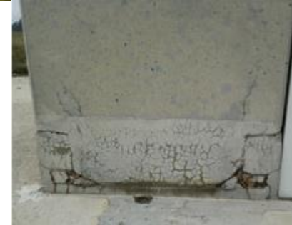
Figure 3: Damage caused by vibrations and at the Lichtenegg Research Park.
