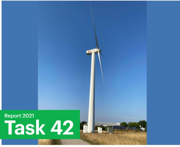
Picture of the DTU V-52 research turbine, which has been chosen as case turbine for estimating the remaining useful life time of older onshore wind turbines based in turbine instrumentation data as well as aero elastic models. The DTU V-52 research was installed at the DTU Risø campus in 2015, but the Vestas V-52 turbine was introduced to the marked in year 2000 and is therefore a typical turbine model that will operate beyond the design life time in the coming years.
