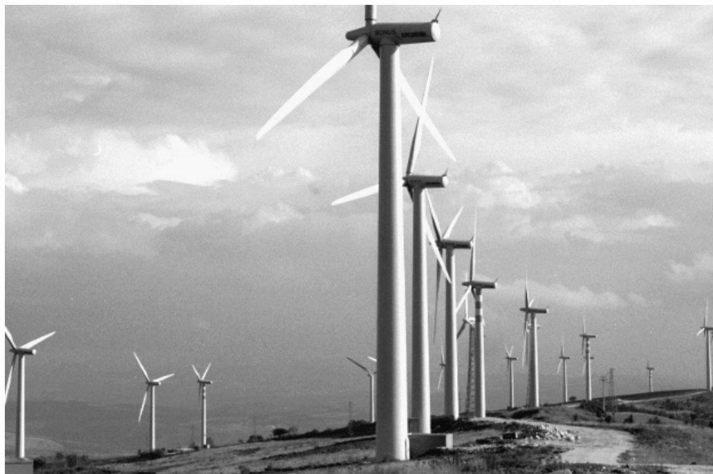
Figure 15.6 Filippo Sanseverino windfarm at Castelfranco in Miscano (2 wind turbines Vestas 600 kW and 48 Bonus 600 kW)
