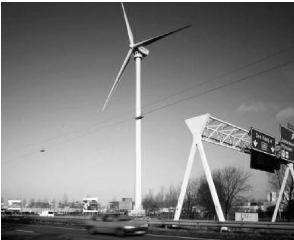
Figure 18.4 Enron-Tacke 1.5 MW with rotor 70.5 m with view platform just under the nacelle
