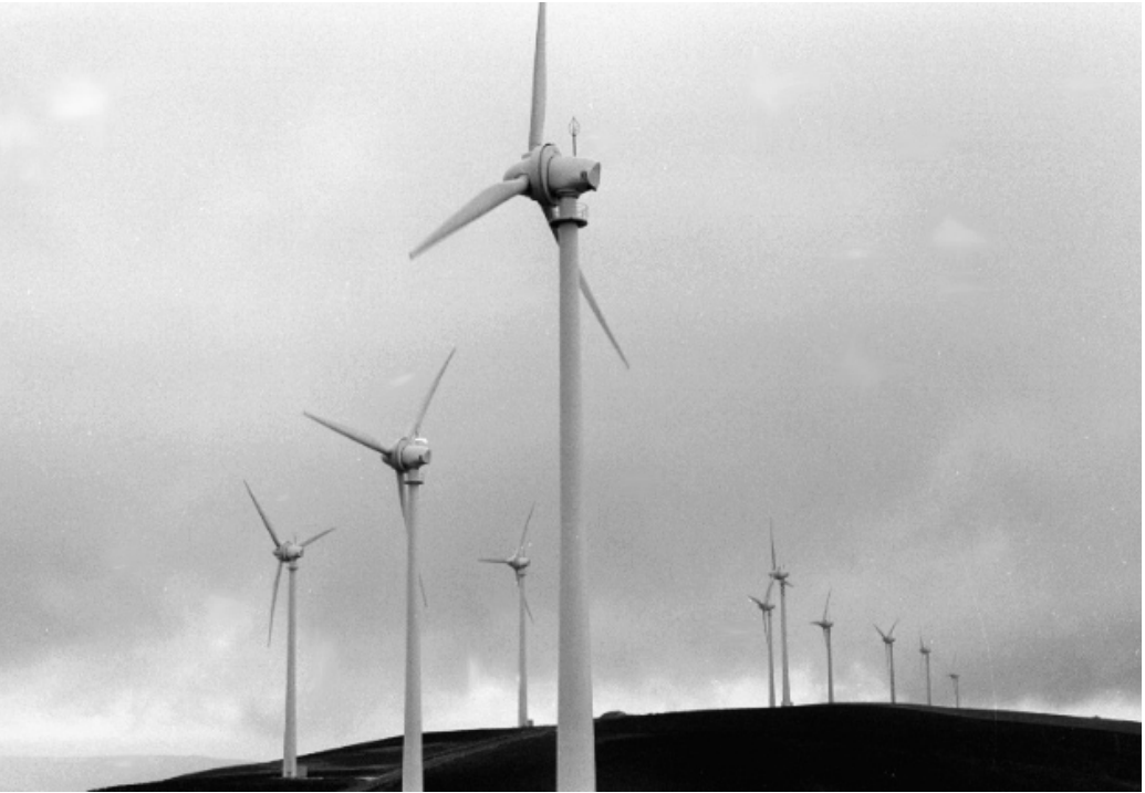
Figure 15.4 Edison Energie Speciali 10 MW windfarm at S. Giorgio la Molara (20 wind turbines Enercon 500 kW)
