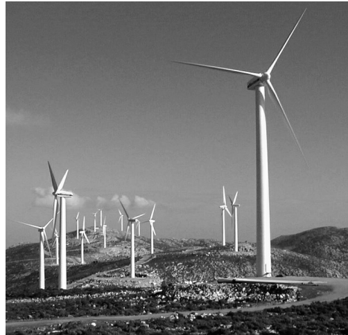
Figure 14.4 Windfarm with capacity of 11.2 MW on Evia Island, comprising 17 Vestas V42, 600-kW wind turbines (provided by G. Gilinou, CRES)
