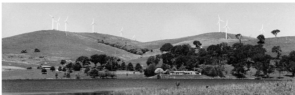
Figure 9.2 Blayney wind farm, New South Wales
