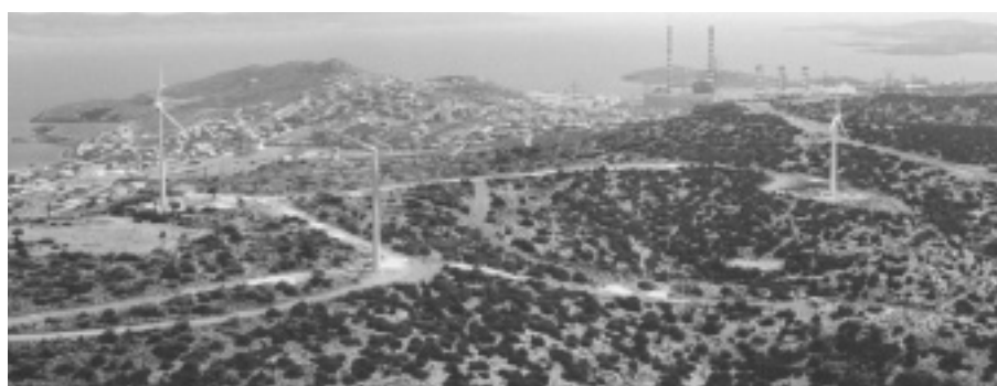
Figure 13.5 CRES's 3.1-MW wind farm located in Lavrio
