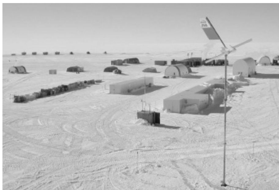
Figure 14.8 The 5-kW direct drive turbine with P.M. generator especially developed for Antarctic environment. Photo at Dome C., Courtesy of National Research Project in Antarctica.
