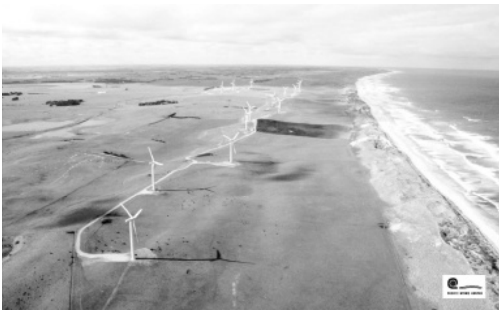
Figure 8.3 Pacific Hydro's 18.2-MW Codrington Wind Farm in Victoria
