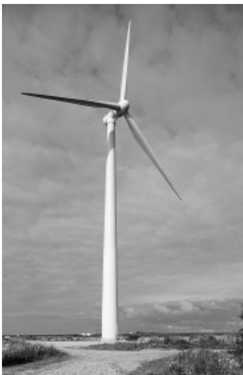
Figure 11.2 WinWinD's 1-MW prototype in operation in Oulu
