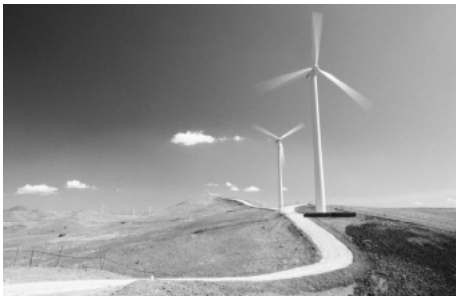
Figure 14.6 View of the 7.3 MW wind farm, with 11 IWT V47 units of 660 kW, which has been built by Enel GreenPower at a hill site near Carlentini in Sicily (photo Carmine La Fratta).
