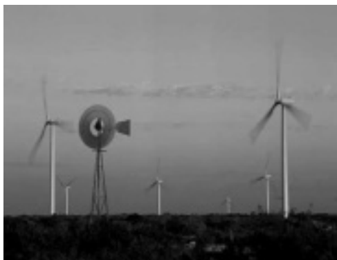
Figure 23.2 Enron Wind 1.5-MW turbines in 150-MW Trent Mesa wind power plant located near Sweetwater, Texas
