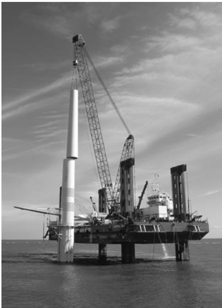
Figure 10.1 Tower construction offshore in Ireland (Courtesy of Airtricity)
