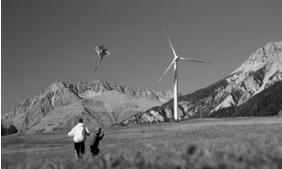
Figure 11.5 Prototype Leitwind 1.2 MW, installed at Malles/Mals in South Tyrol/Alto Adige
