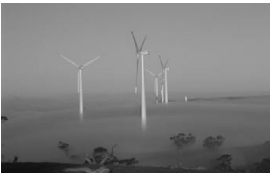
Figure 4.2 Mist below Chalicum Hills wind farm during construction Image courtesy Keppel Prince
