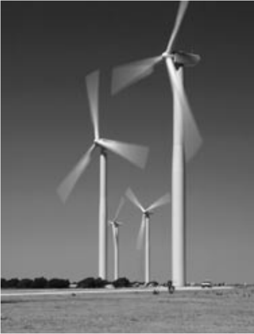
Figure 21.4 New Mexico wind farm that contains 136 GE wind turbines of 1.5 MW and contributes 204 MW to the national wind energy capacity
