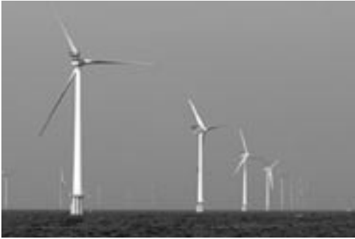
Figure 6.4 Offshore wind farm at Horns Rev, 160 MW
