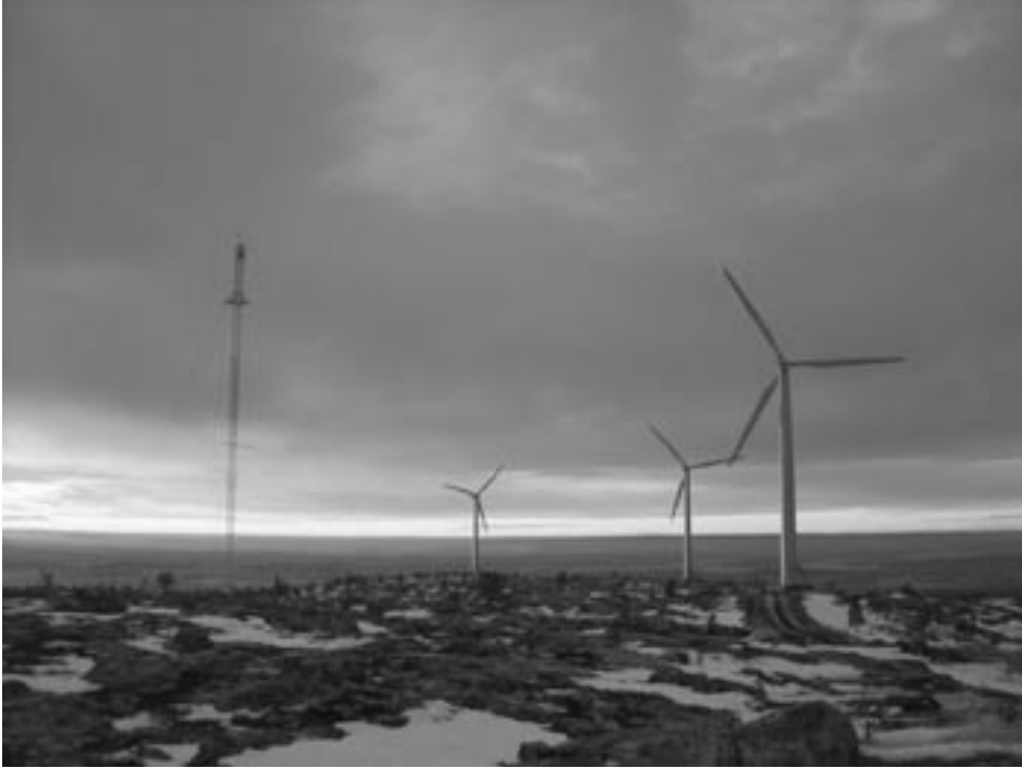
Figure 2.5.2 Long-term measurement campaign including monitoring of adapted technology suitable for severe icing climate has been carried out since 1999 at Olostun-turi-fjeld wind farm
