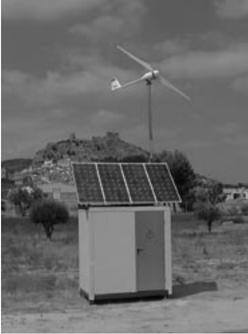
Figure 17.10 Hybrid system for an isolated application
