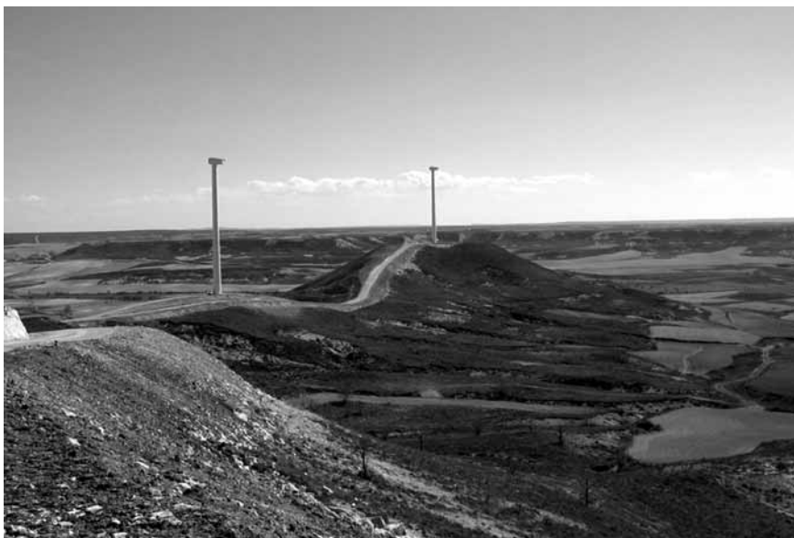
Figure 6 Wind farm under construction in Castilla-Leon.
