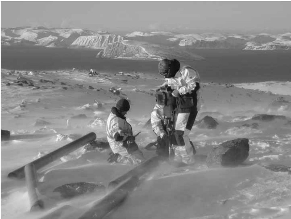
Figure 1 Foundation work in connection with site measurement campaign. Photo: Kjeller Vindteknikk, Norway.
