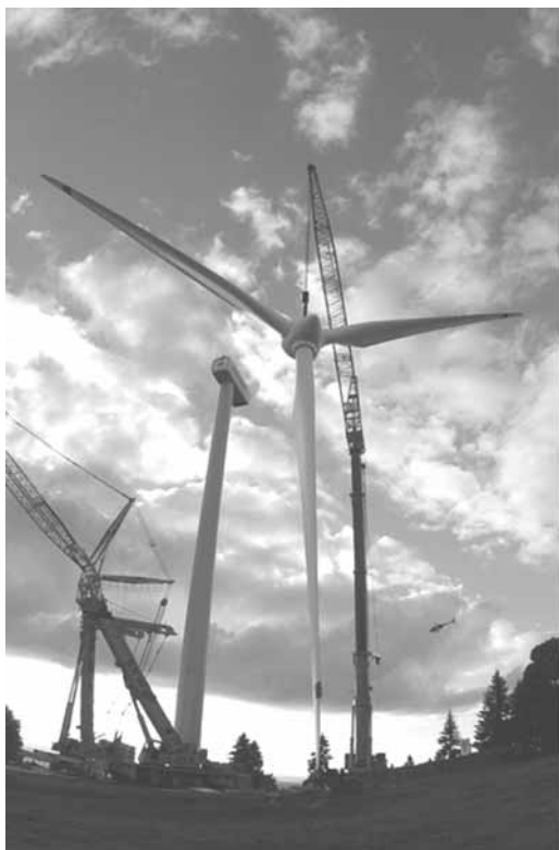
Figure 2 Installation of a 1.75-MW wind turbine on Mt. Crosin by Juvent SA.
