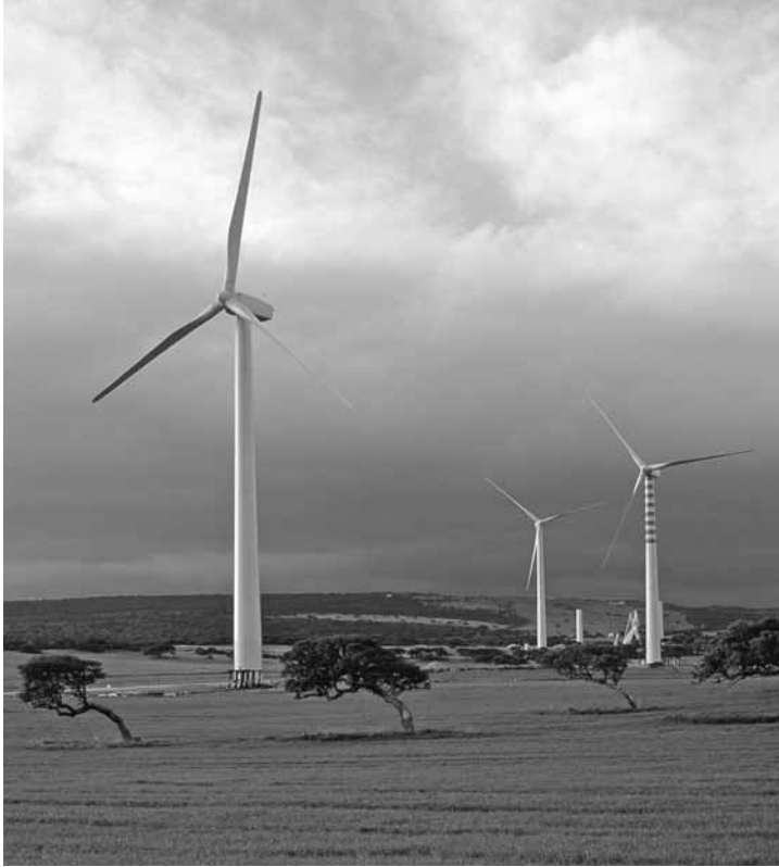
Figure 4 GE Wind 1.5-MW turbines at Enel GreenPower's site of Littigheddu (Sardinia).
