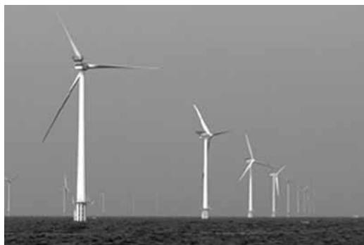
Figure 4 Offshore wind farm at Horns Rev, 160 MW. Published with the permission of ELSAM.
