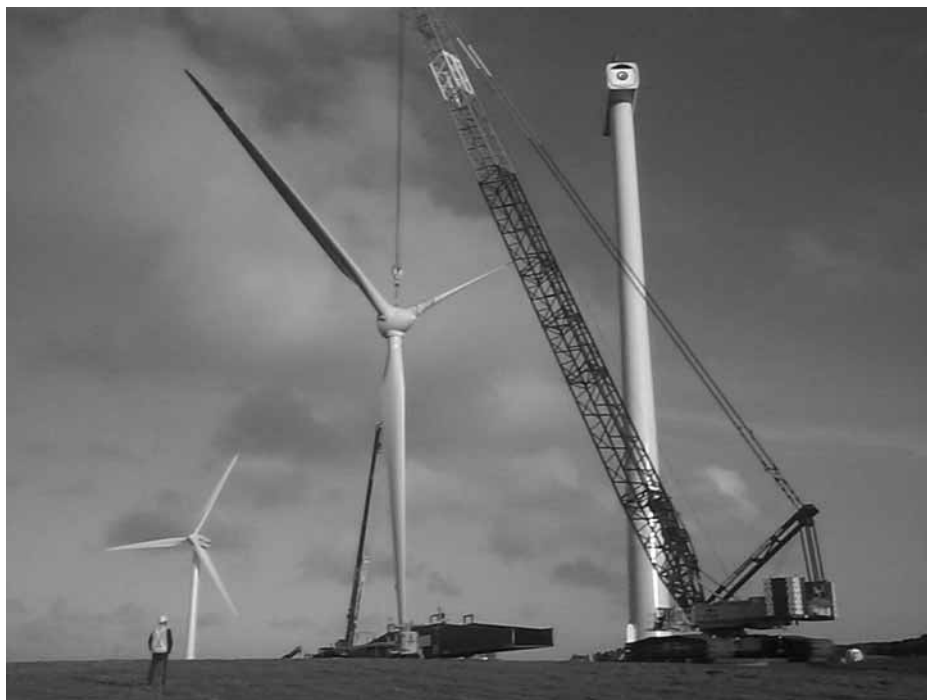
Figure 5 Construction at Woolnorth Wind Farm, Tasmania.
