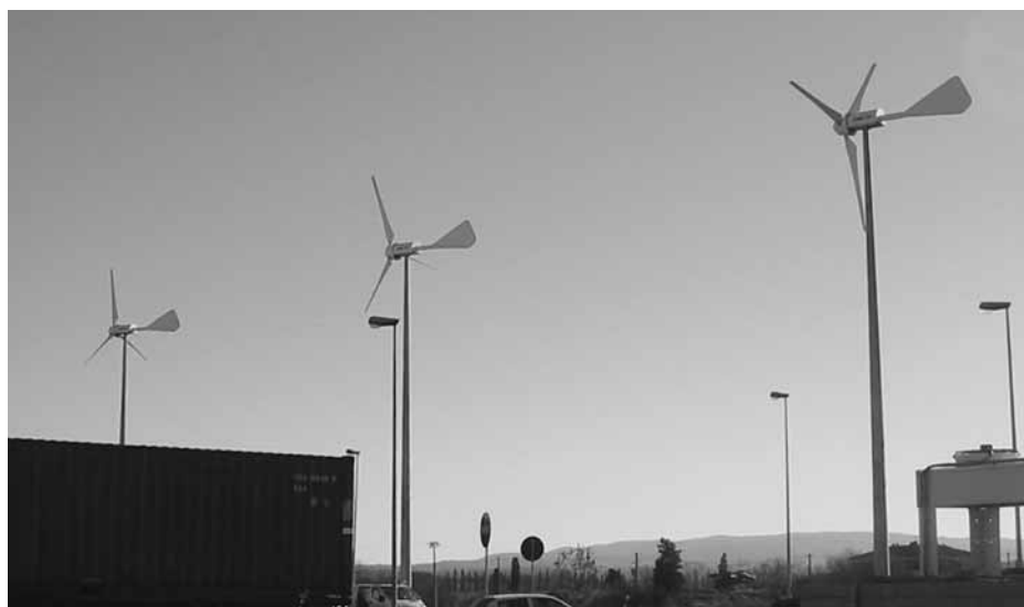
Figure 6 JIMP 20 small turbines (20 kW) developed by Jonica Impianti.
