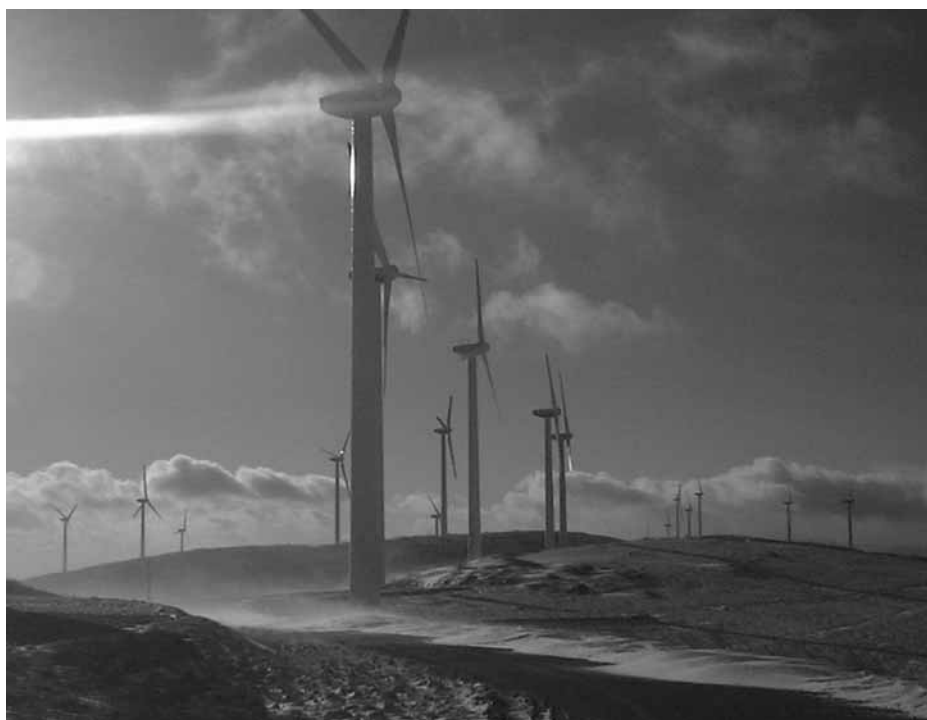
Figure 3 In 2004, Urus Energy developed the largest wind farm in Japan at Kamaishi, Iwate. Power output is 42,900 kW from 43 units of 1-MW Mitsubishi Heavy Industries Ltd. wind turbines.
