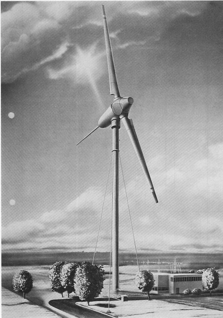
Fig. 1: Large Wind Energy Plant GROWIAN
