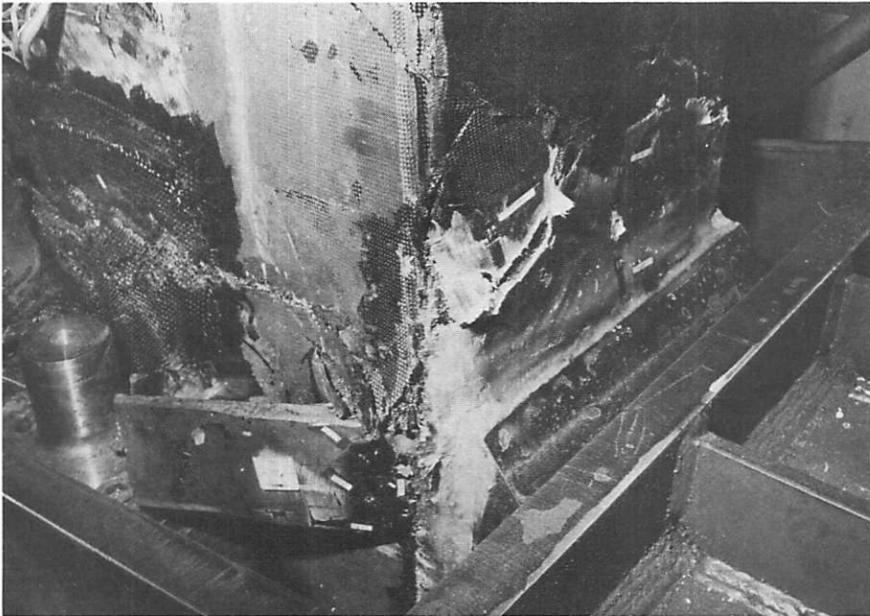
FIG. 14: Failure in the web
