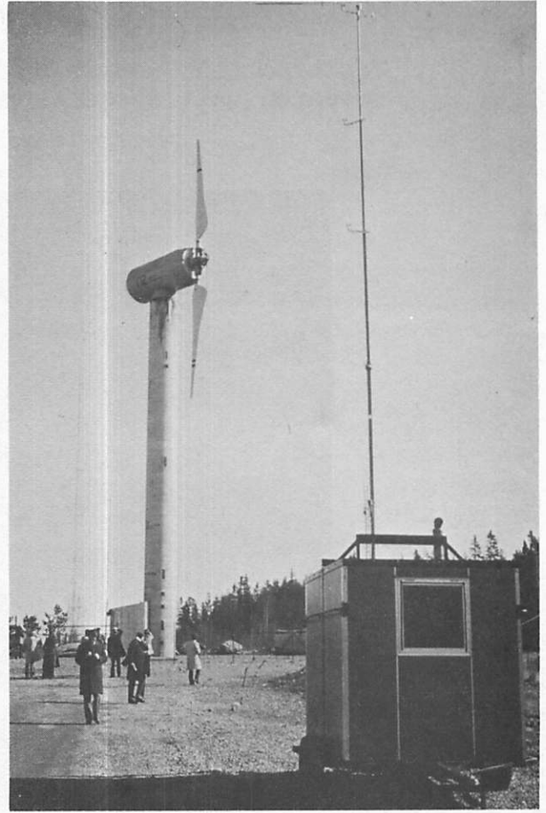
The 60 kW unit
