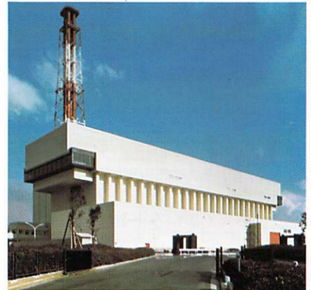
ITABASHI Incinerator Plant, Tokyo, Japan. Capacity 1200 TPD (Metric)
