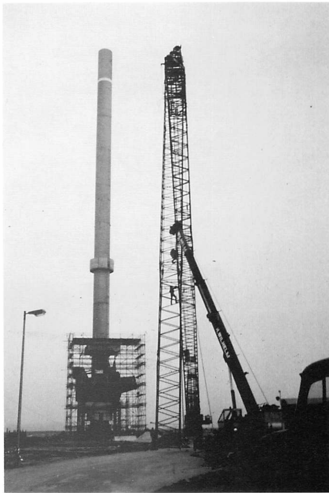
Fig. 3: Middle section of nacelle lifted over the base of the tower
