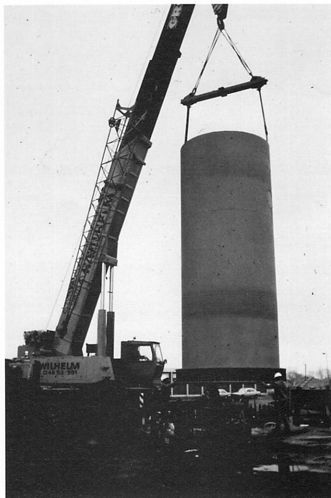
Fig. 1: Erection of first section of tower
