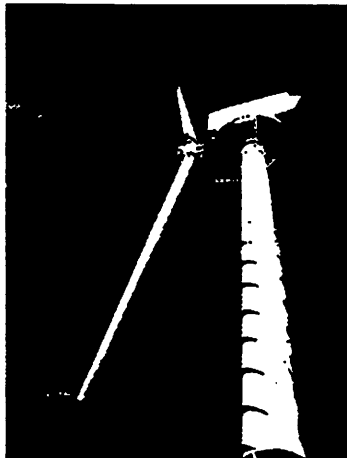
Figure 12. AWT-26 300 kW Utility Turbine
