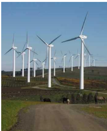
Carballeira Wind Farm - Spain
