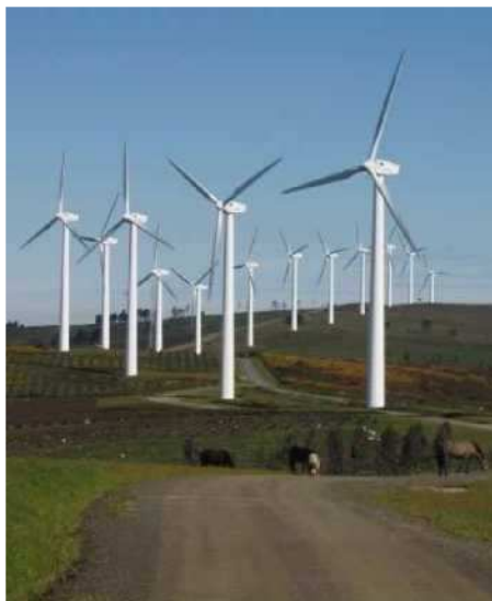
Carballeira Wind Farm - Spain
