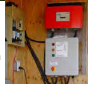
2.5-kW turbine and single-phase inverter for net-metering applications
