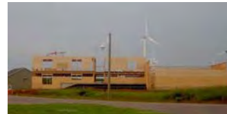
WEICan under construction
