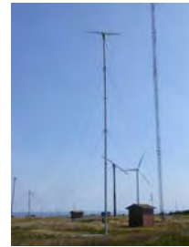
Bornay 3 kW turbine in single-phase net metering at WEICan
