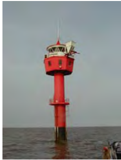
Sodar application off-shore (picture Ecofys) and within wind farm
