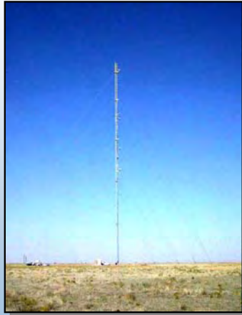
120 meter meteorological mast south of Lamar, Colorado
