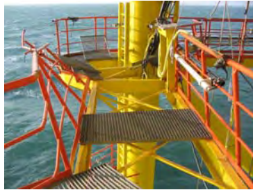
Storm damage on lower platform, C.D. + 14.5 m
